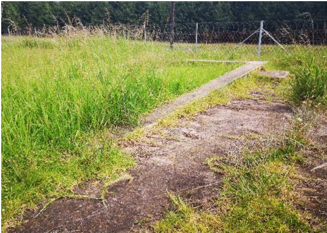
Figure 4: Foundations of structure on BESS facility site
