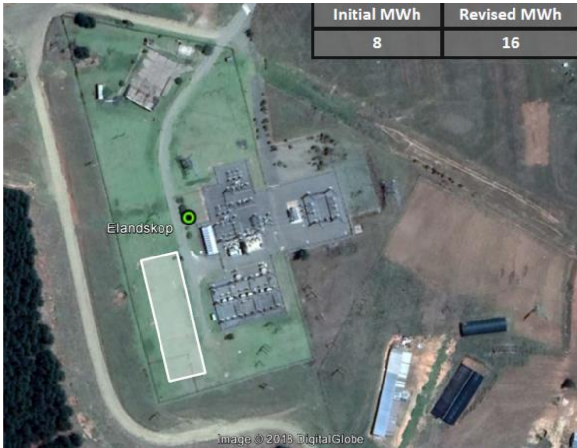
Figure 3: Elandskop substation with proposed BESS site depicted in white (1World Consultants)
