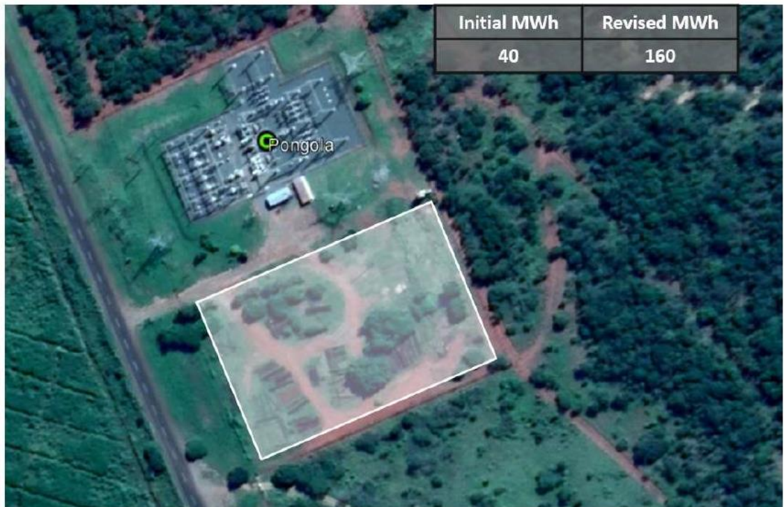
Figure 3: Pongola substation with proposed BESS facility depicted in white (1World Consultants)
