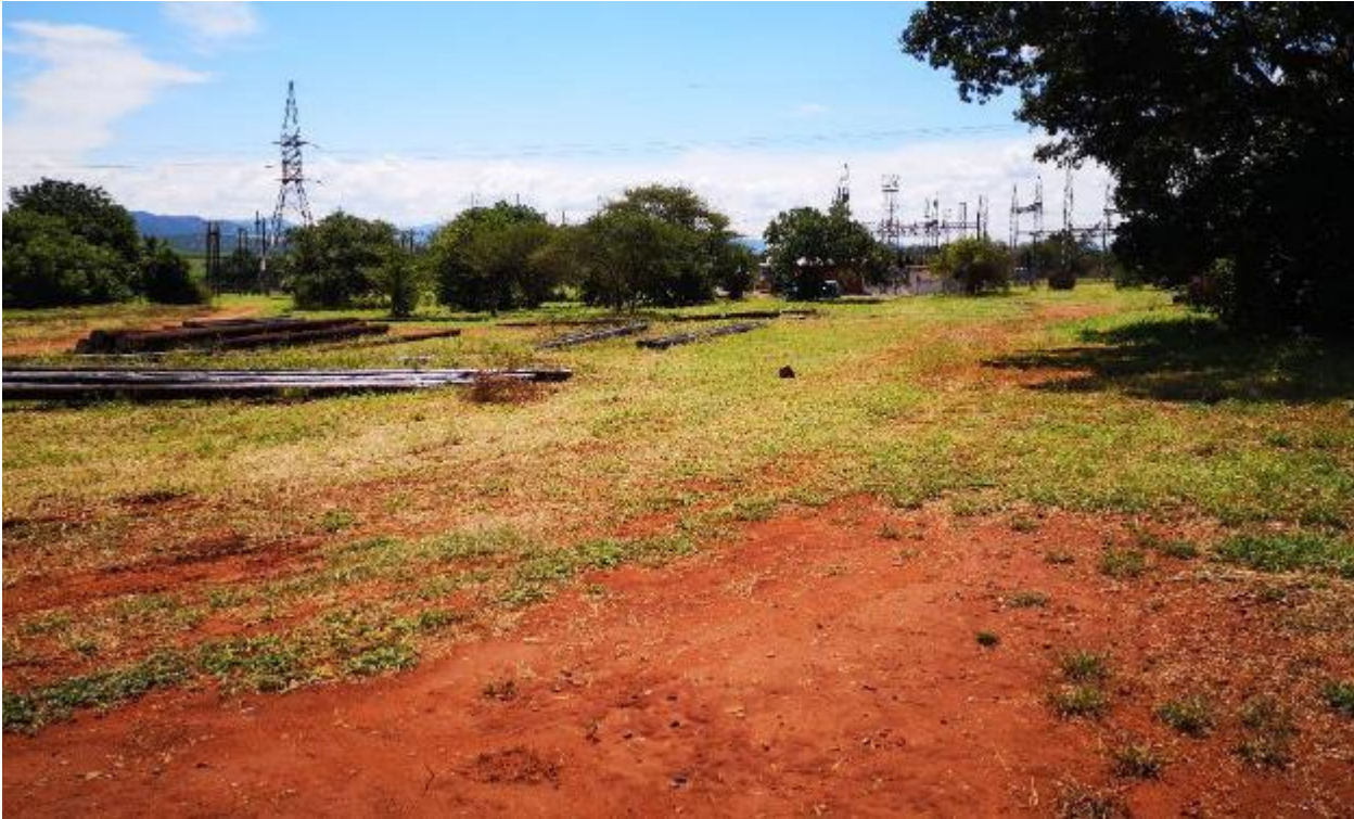
Figure 5: View towards substation which will be developed for BESS facility
