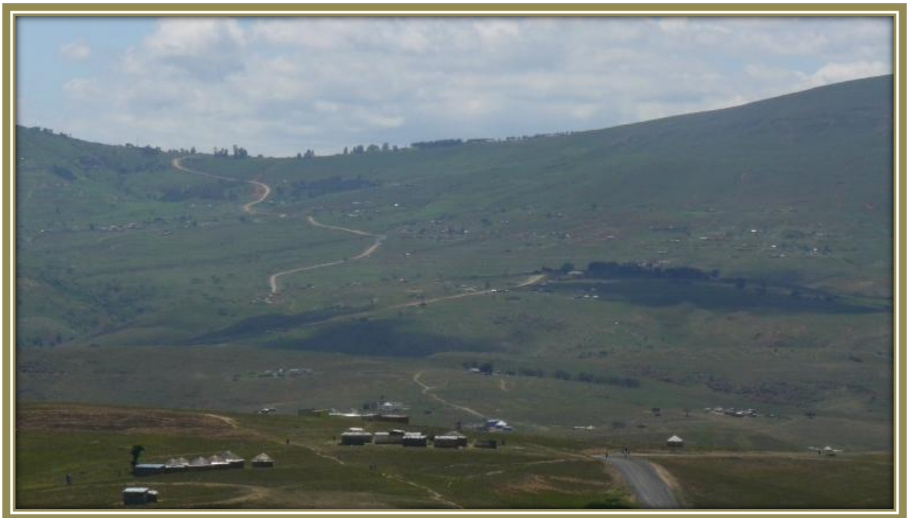
Pipeline alignment within road reserve
