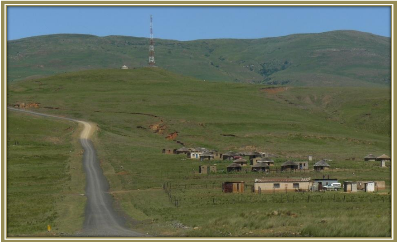
Existing infrastructure within road reserve – (note yellow water line marker)
