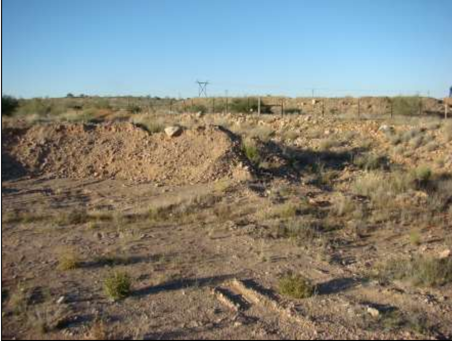
Fig.3 Soil works at existing waste disposal site at Keimoes, Northern Cape.
