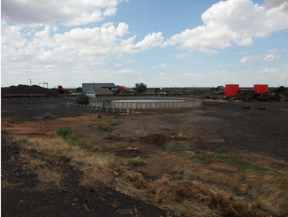
Figure 5: View indicating the disturbance.
