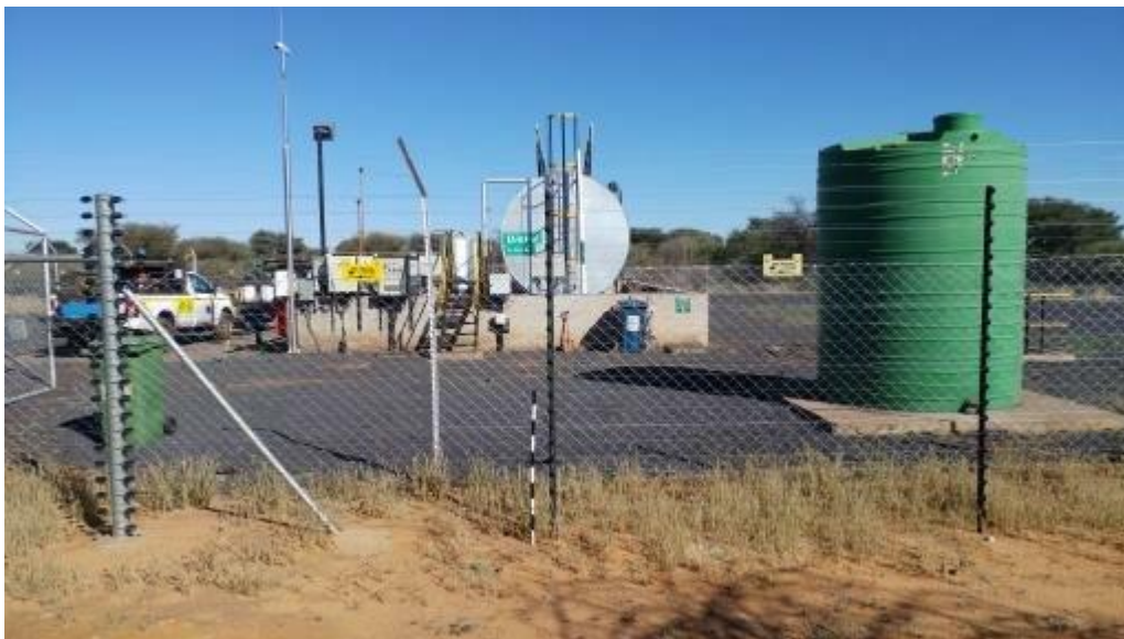
Figure 8: View of diesel depot at the preferred location.
