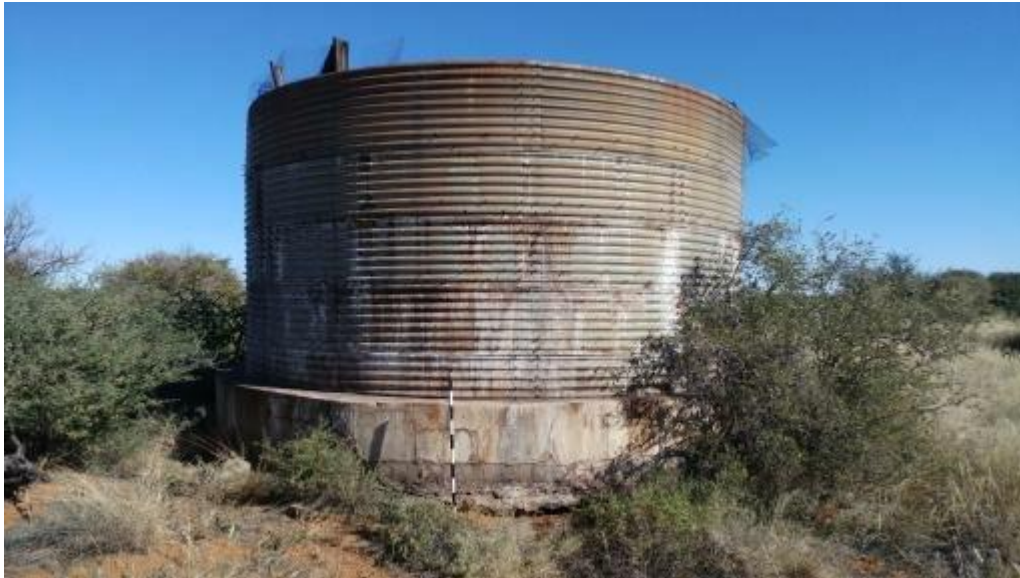
Figure 7: View of dam at the preferred location.
