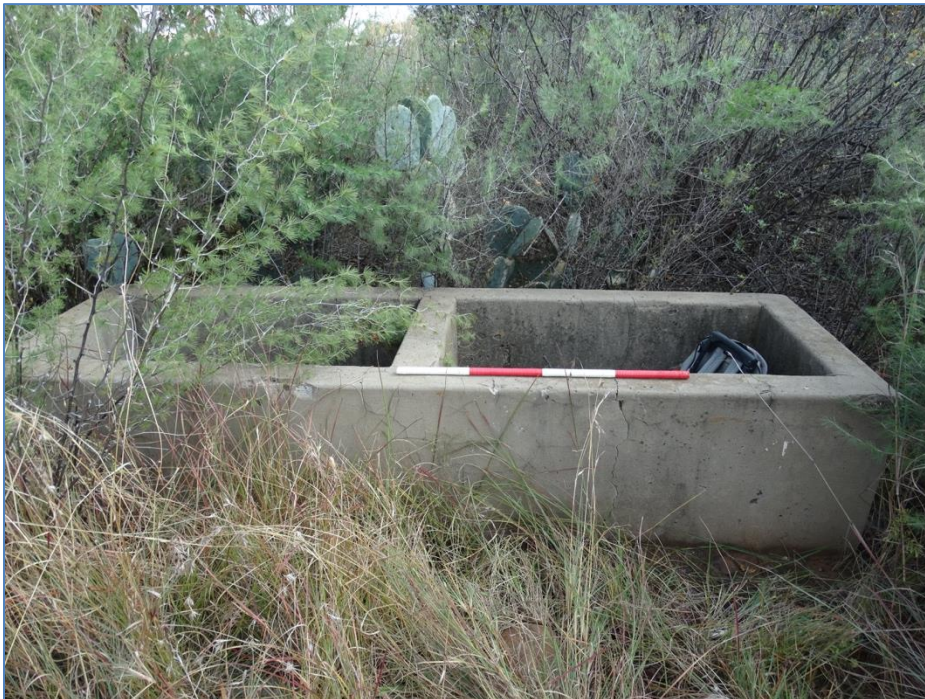
Figure 19. Concrete platform and trough identified at CS1.
