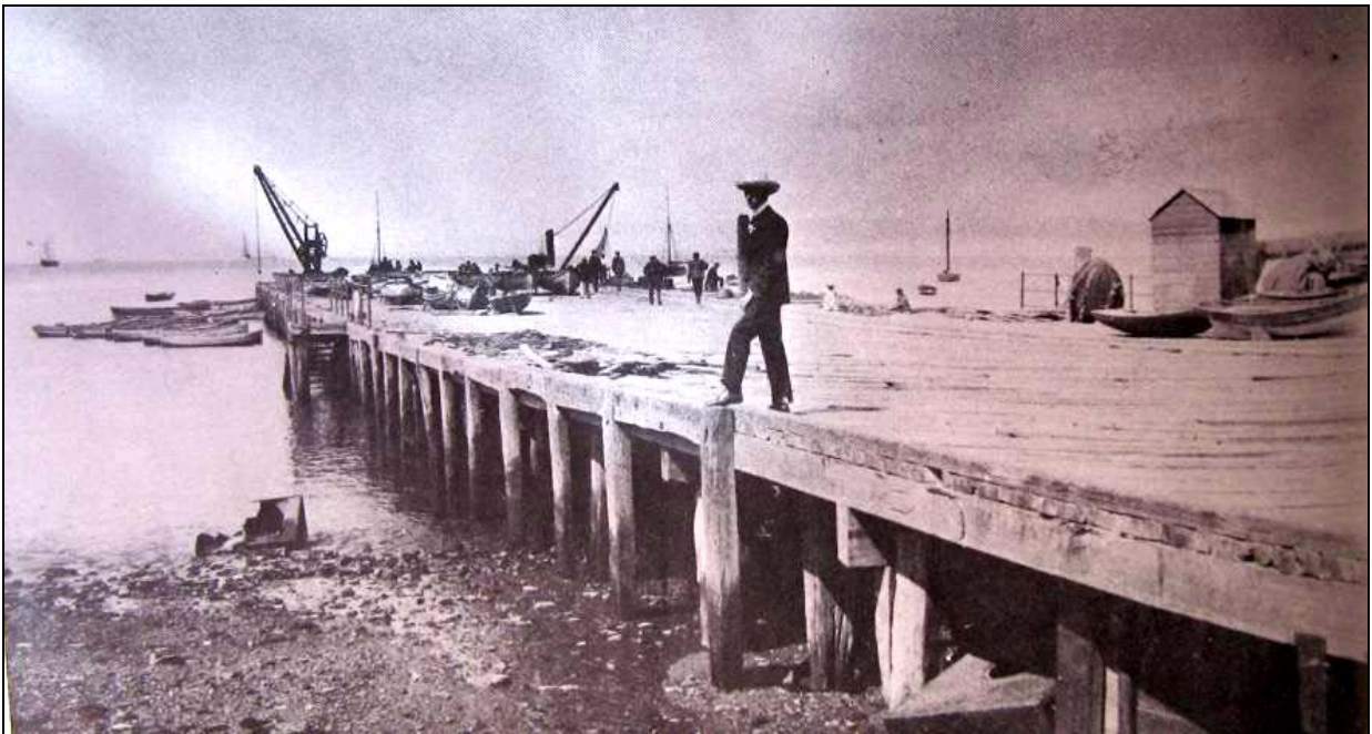
Figure 7: Photograph of the wooden jetty (Central jetty) at the end of Adderley Street c1902 (Picard 1969:118). The central jetty was constructed in the 1850's and became the central hub of harbour activities. In 1907 the jetty was extended to create a central pier and promenade. The pier was demolished in 1938 to make way for the Foreshore Reclamation Scheme (Patrick et al 2010). M4/12 c1910 shows the extent of the land reclamation as well as a dashed line to the NE of the Customs House – possibly showing the outline of the earlier wooden jetty.
