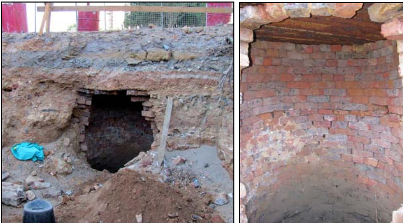
Plate 10: The damaged side of the well showing overburden.
