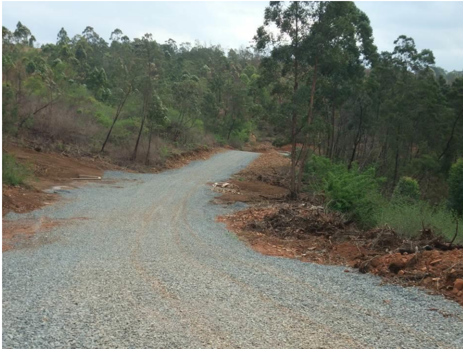
Figure 8: Section of road that will be upgraded.
