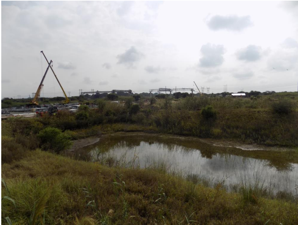
Figure 8: Another view on site.
