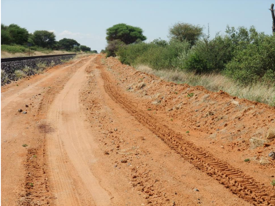
Figure 7: Another view along the proposed railway alignment.
