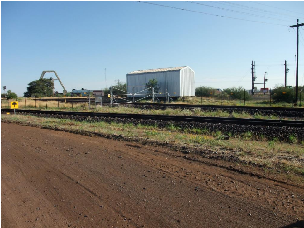
Figure 4: General view of the current railway and servitude close to Gloria Mine.
