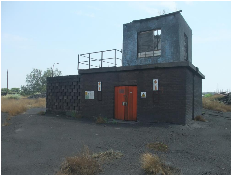
Figure 17: Building used for power generation when the plant was in operation.
