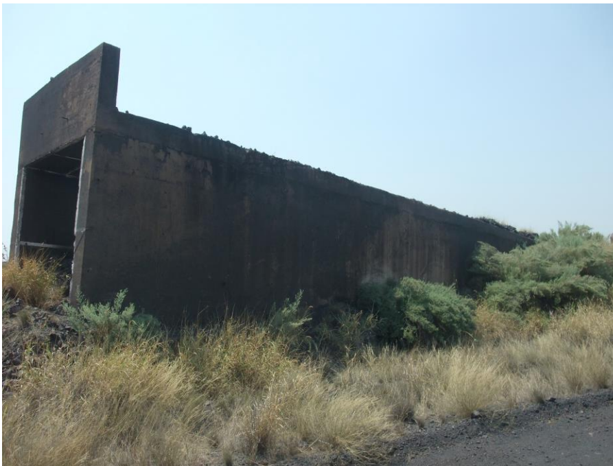
Figure 19: Side view of the above structure.
