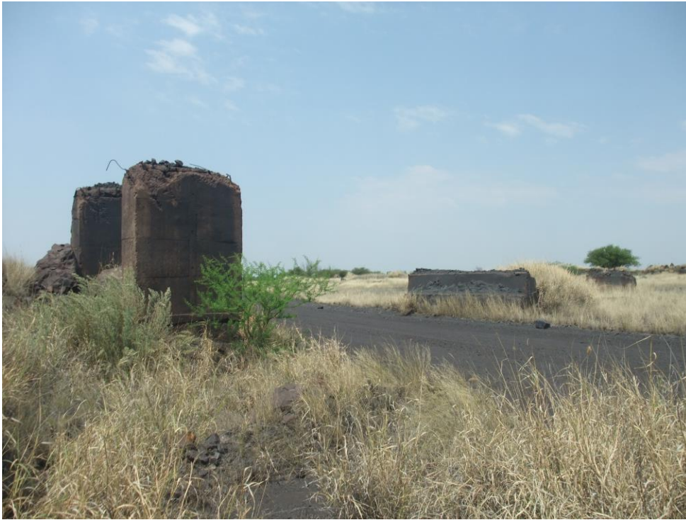
Figure 20: Section of a bridge in the study area.
