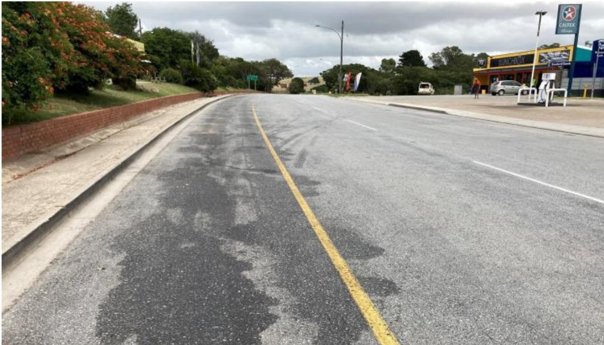
Figure 12: Another view along the road indicating the disturbance around the road
