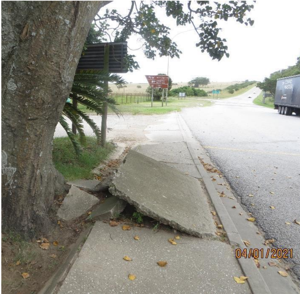
Figure 9: Note sidewalks and grass indicating a landscaped environment along the route
