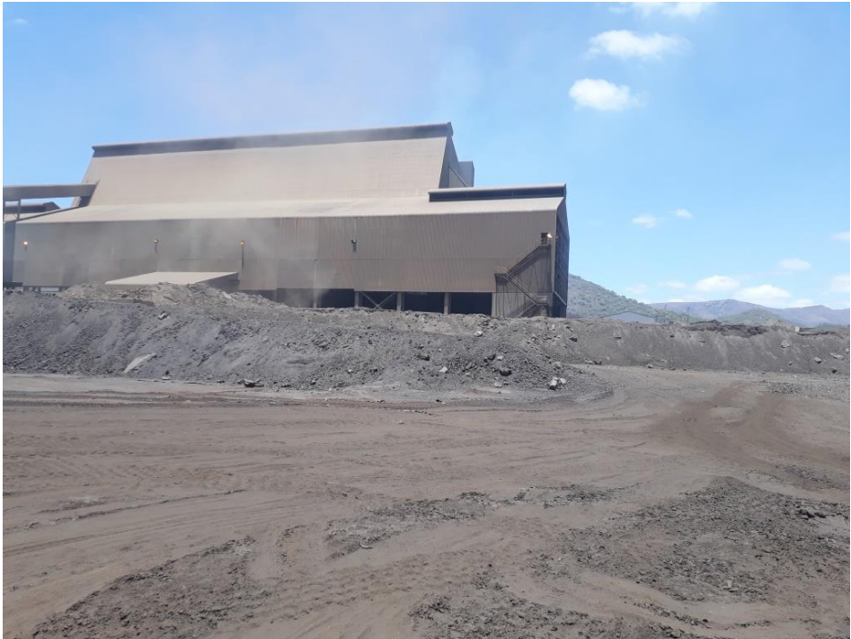
Figure 16: Another view at site 2.
