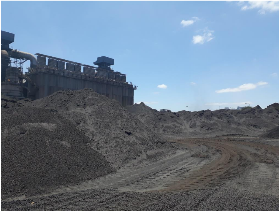
Figure 12: Another view at site 1.
