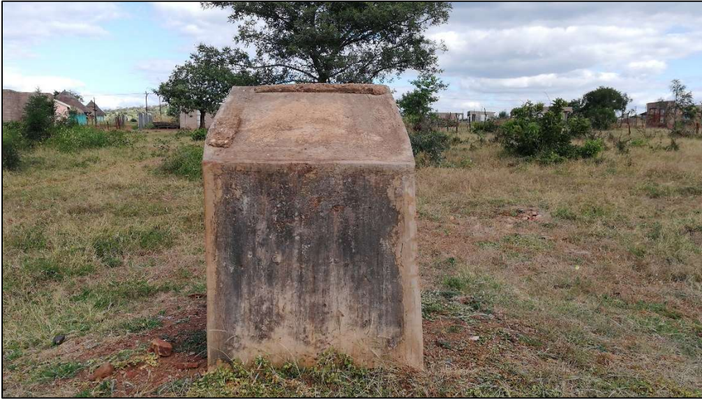
Figure 31: Pedestal of rehabilitated shaft.
