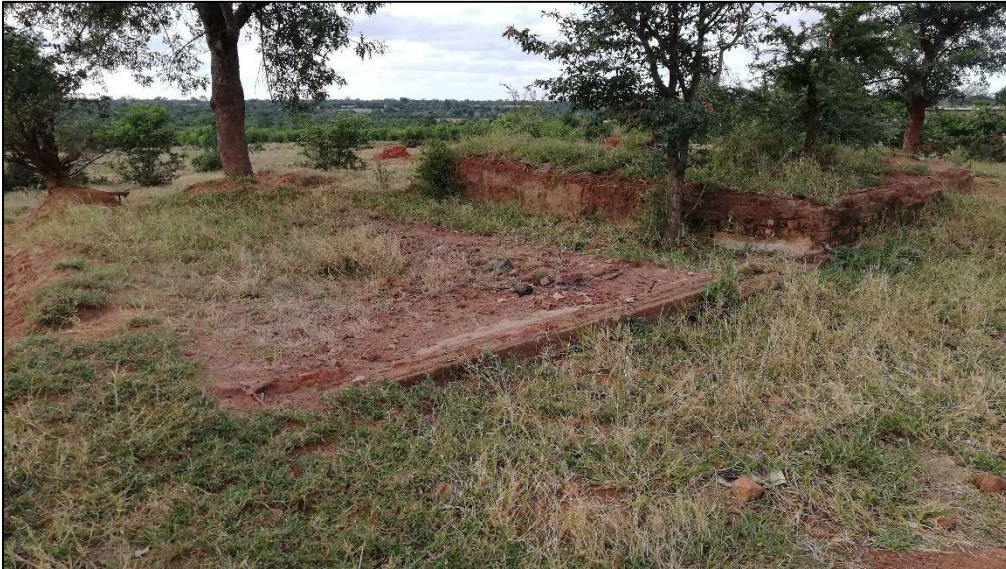
Figure 29: Building foundations at proposed Pit 06.
