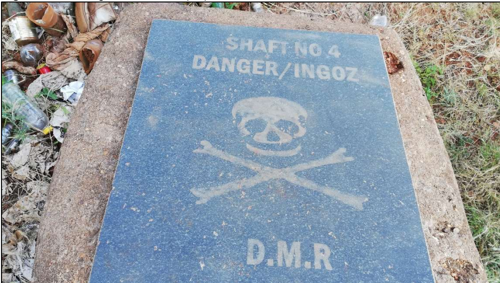
Figure 30: Granite top of rehabilitated shaft No 4.
