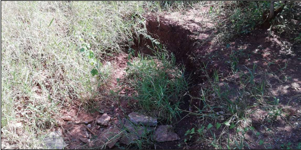
Figure 25: Pieces of concrete at proposed Pit 05.
