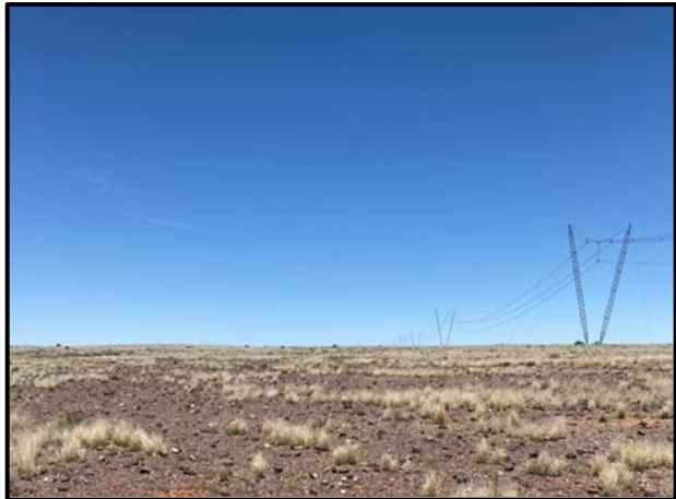
Figure 4.2. Existing powerline in the southern section of the study area.
