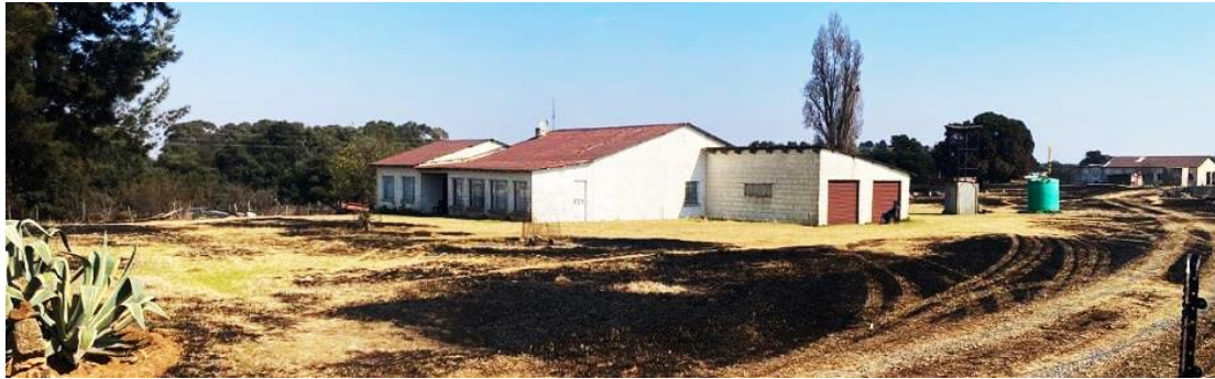
Figure 25. Existing farmstead viewed from the east. (Photo S.U. Küsel 2023.)
