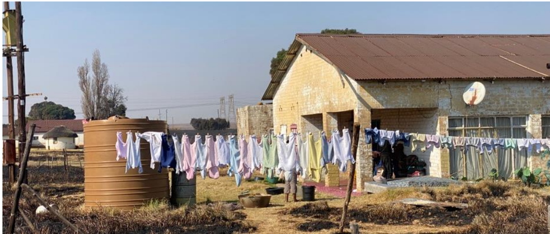
Figure 33. Converted farm shed/ dwelling seen from the west. It is fully serviced with electricity, water and septic tank for waste-water disposal. (Photo S.U. Küsel 2023.)
