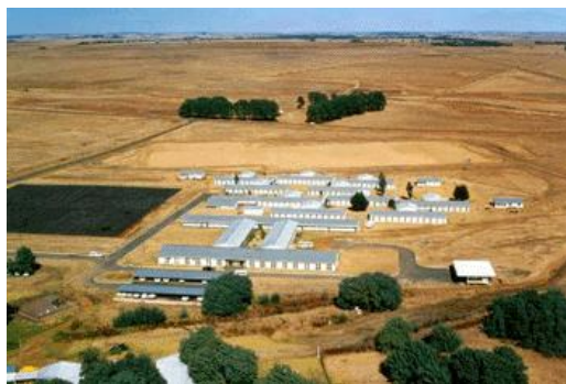
Figure 15. Aerial View of the security training centre at Arnot Power Station.
