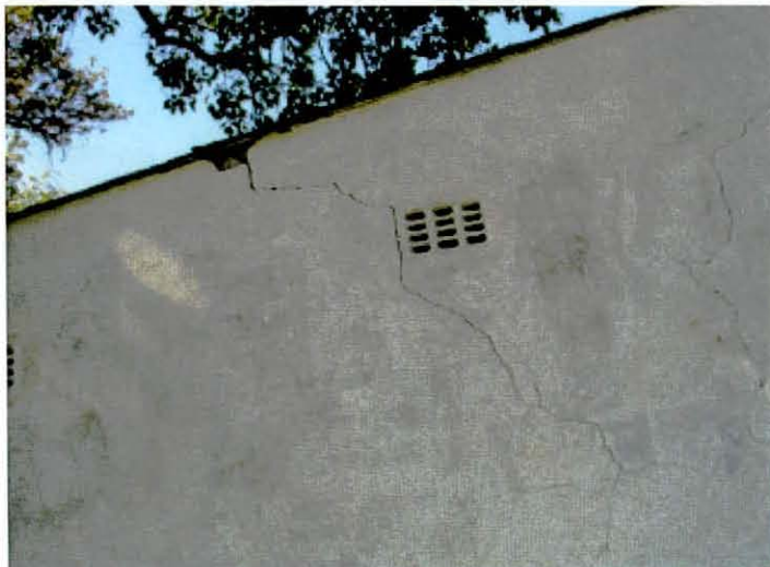
Figure D: Damage as a result of water ingress via unsealed and porous roof timbers
