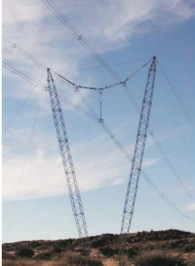
Plate 11: Compact cross rope suspension tower (Pallett, 2009)
