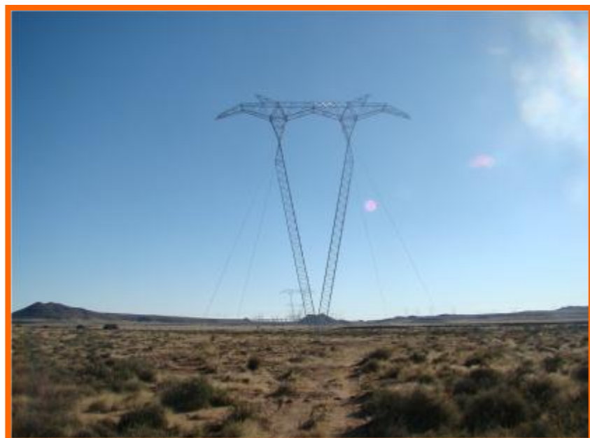
Plate 2: Guyed Vee structure. ((Photography: H. Mlotshwa 2013)
