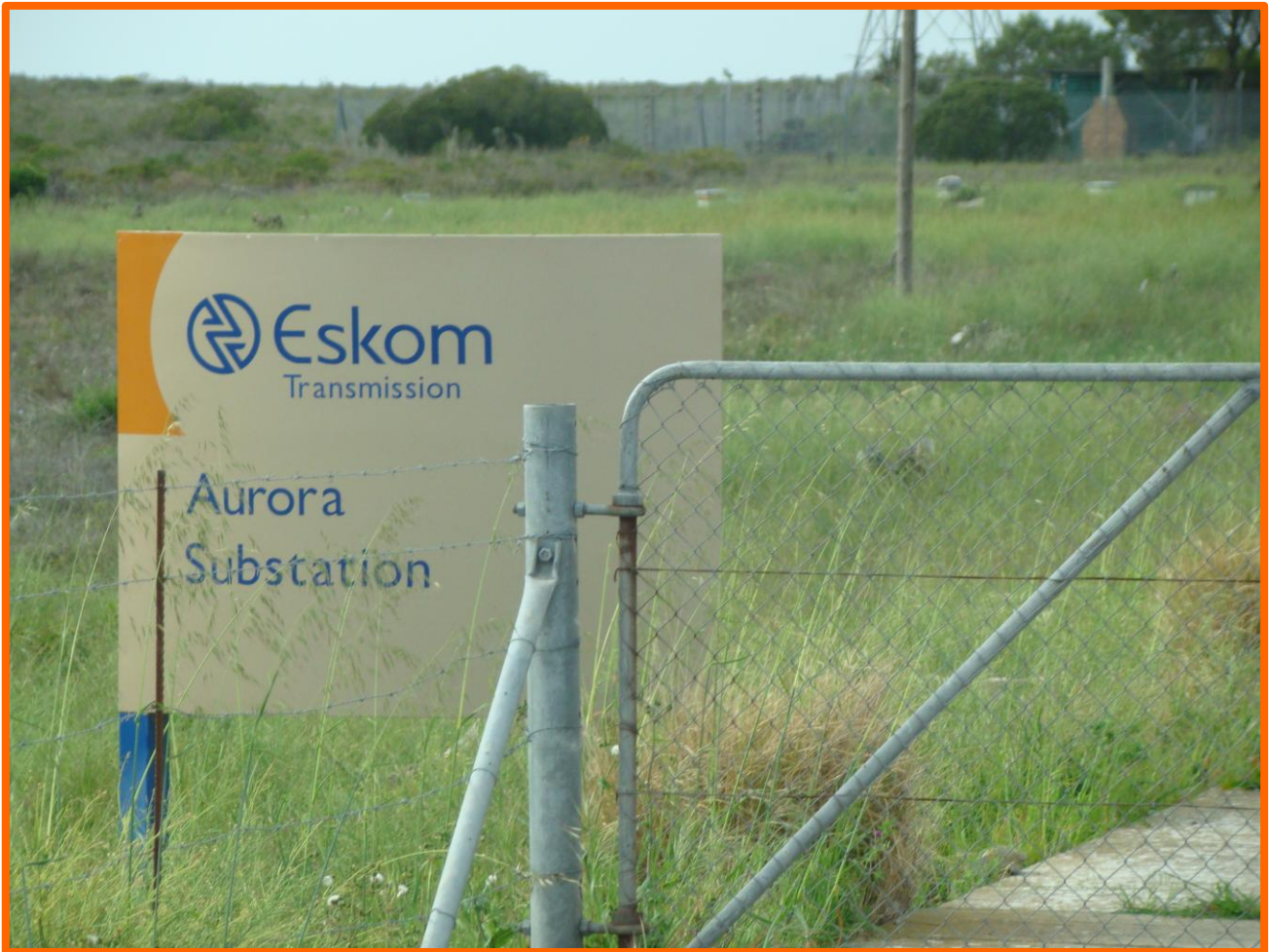
Plate 8:View of existing substation Aurora (Photography: H.Mlotshwa 2013)
