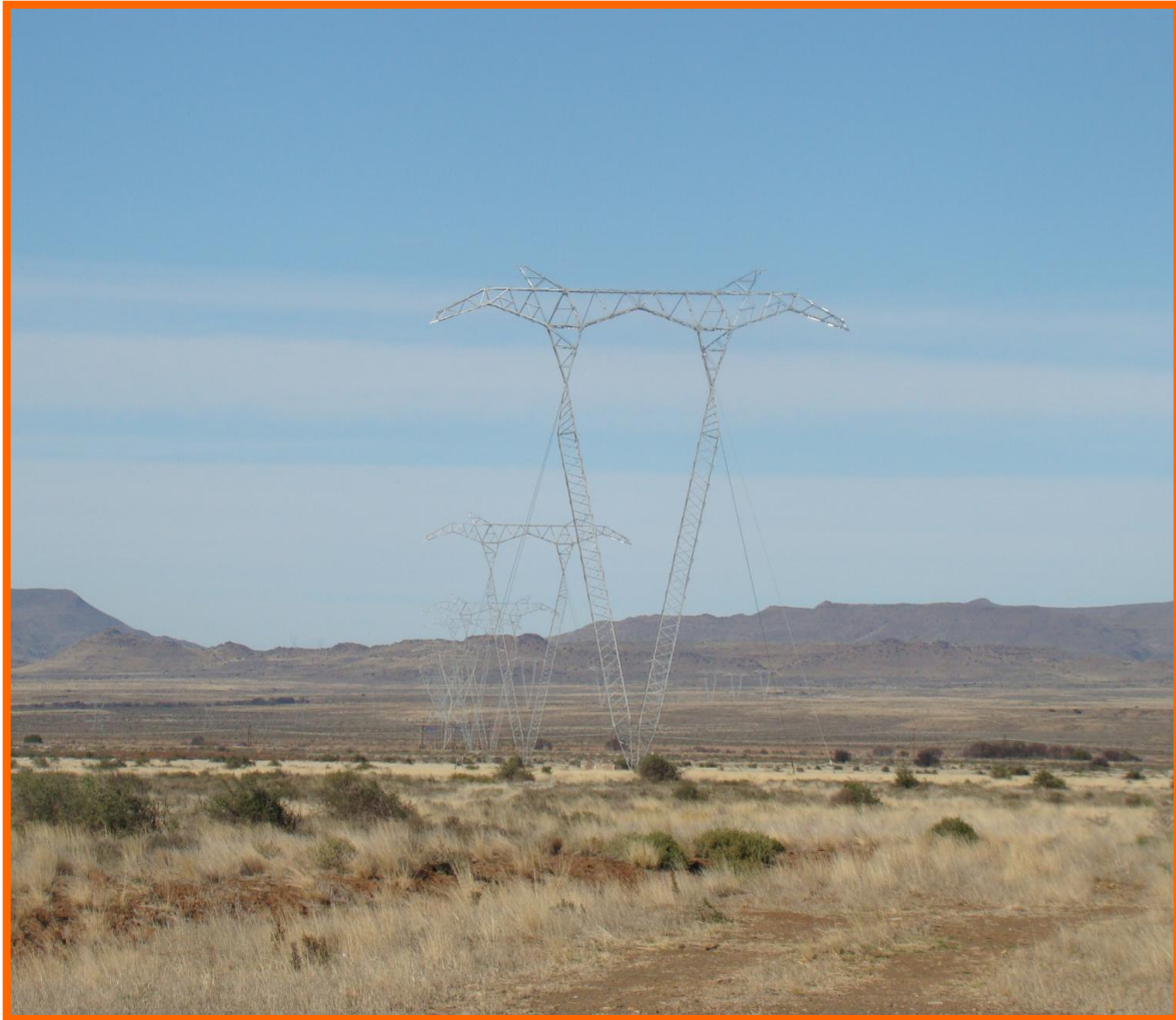
Plate 12: Guyed vee suspension tower (Photography: H. Mlotshwa, 2013)
