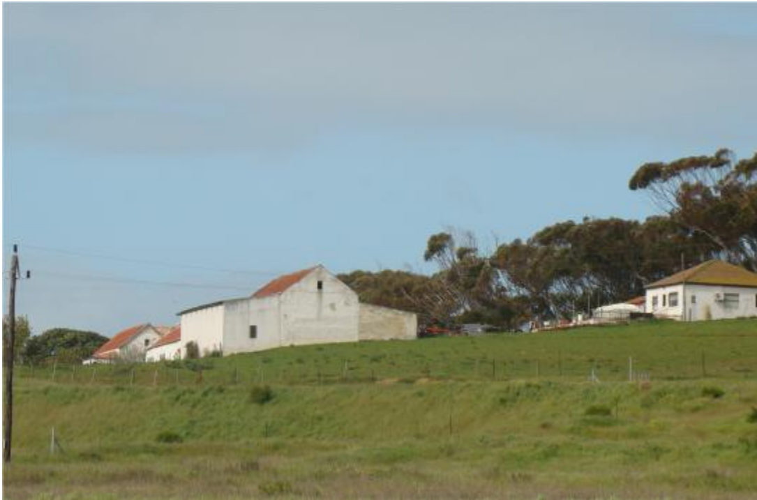
Plate 15: Cape Dutch Houses next to Omega substation
