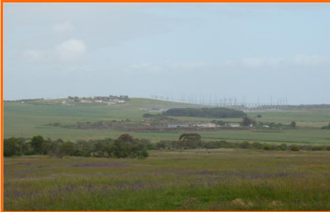
Plate 14: Visual of Omega substation and its surroundings.
