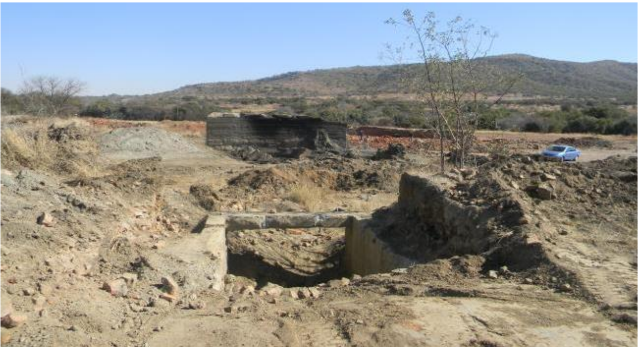
Plate 14: Photo 14: View of vandalized brick moulding infrastructure at the centre of the site (Photograph © by Author 2016)
