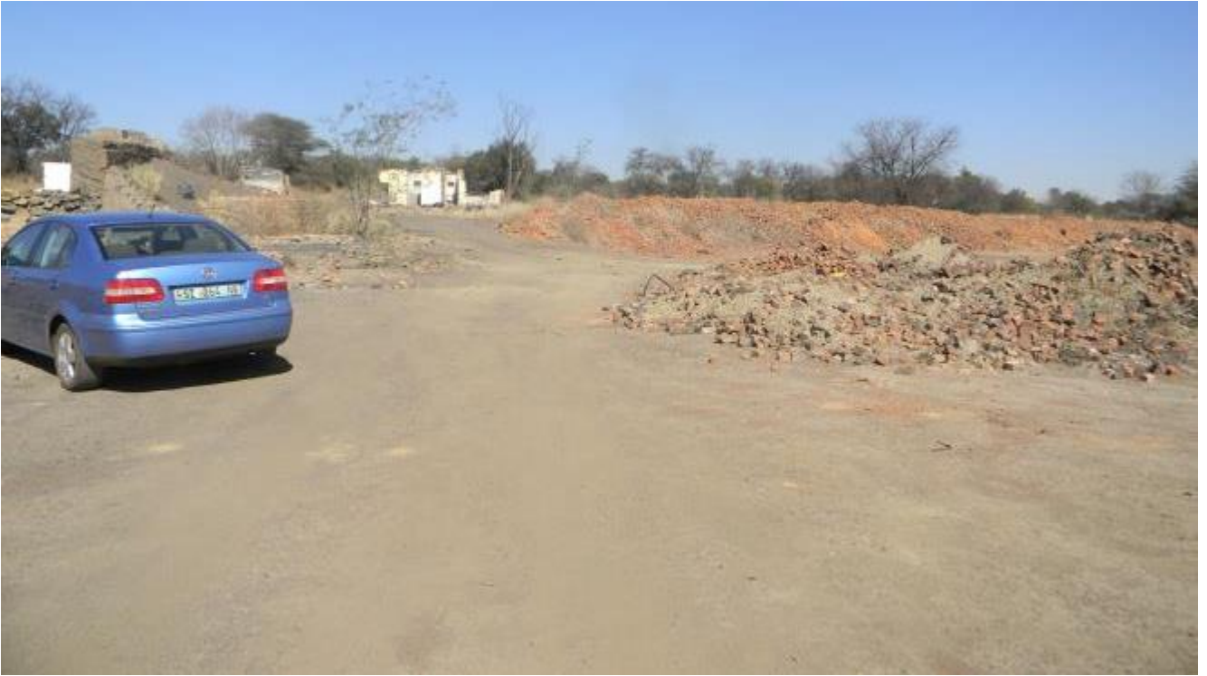
Plate 3: Photo 3: View of dilapidated brick moulding infrastructure including rubble stockpiled all over the site (Photograph © by Author 2016).
