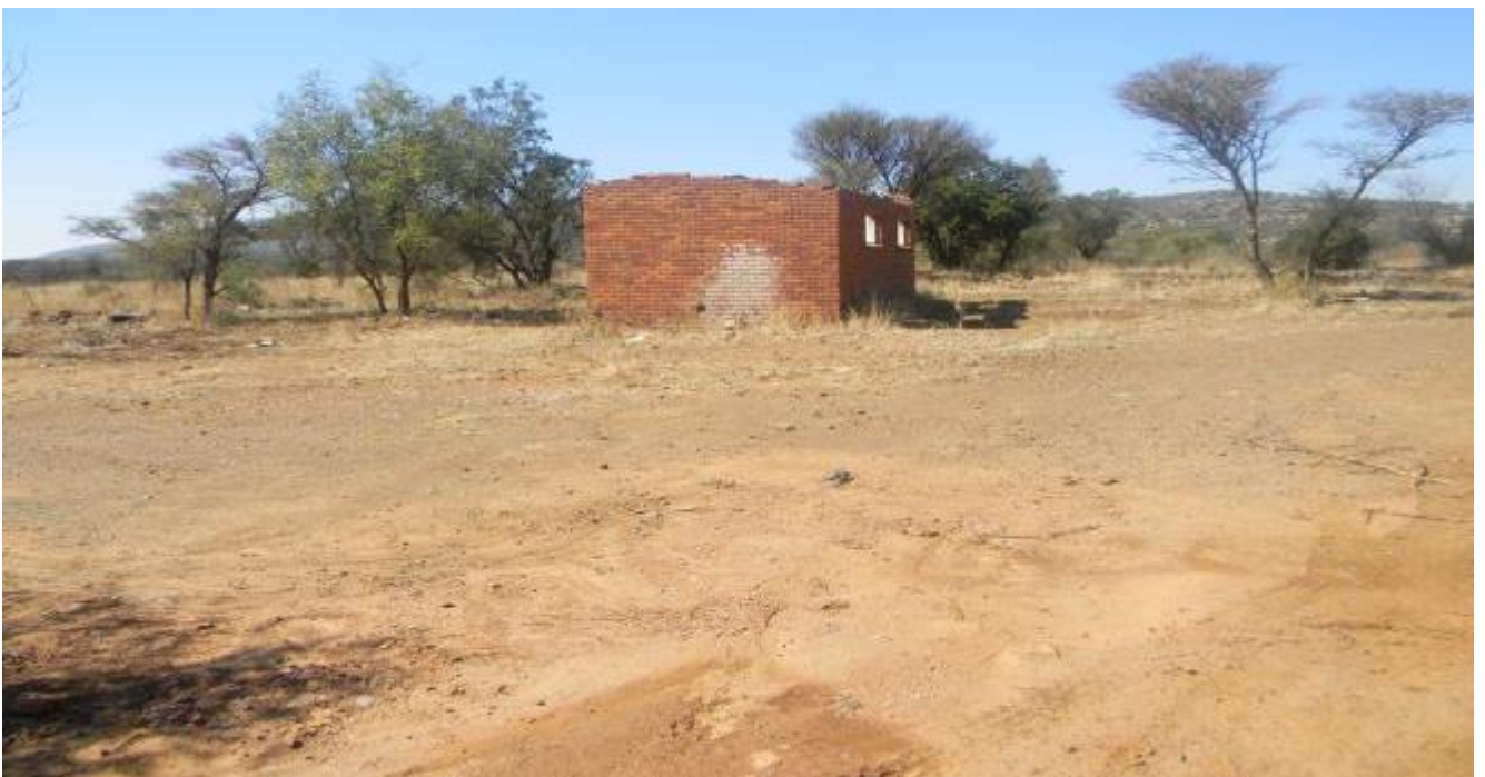
Plate 6: Photo 6: View of remains of an intact structure at the proposed site. Note that such intact structures are targeted by those recovering reusable bricks (Photograph © by Author 2016).
