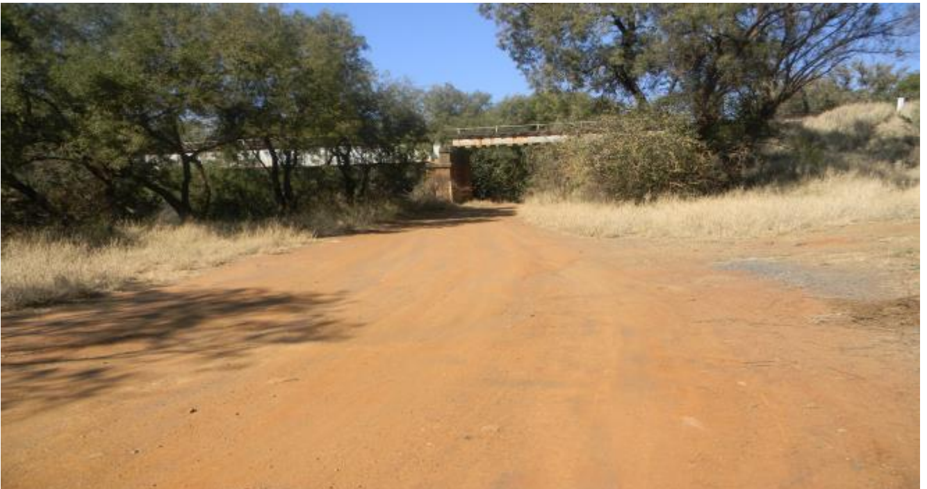
Plate 18: Photo 18: View of an access road that marks the eastern boundary of the proposed development site (Photograph © by Author 2016)
