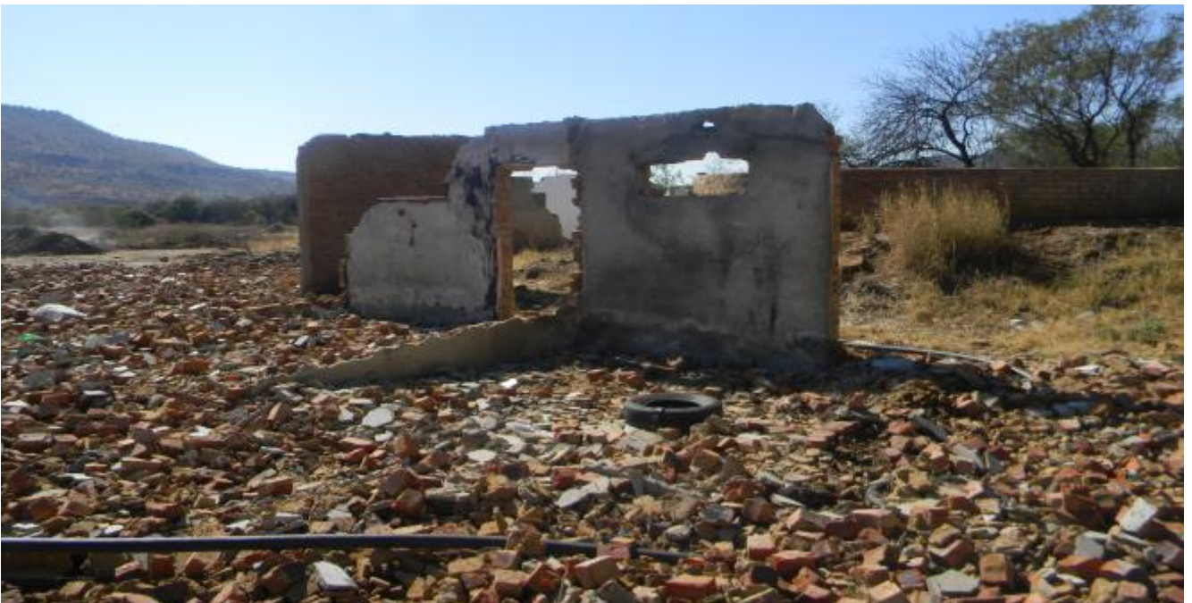
Plate 12: Photo 12: View of ruined brick moulding structures at the centre of the site. Note that these structures are destroyed by members of the local communities salvaging for reusable bricks and still. (Photograph © by Author 2016)
