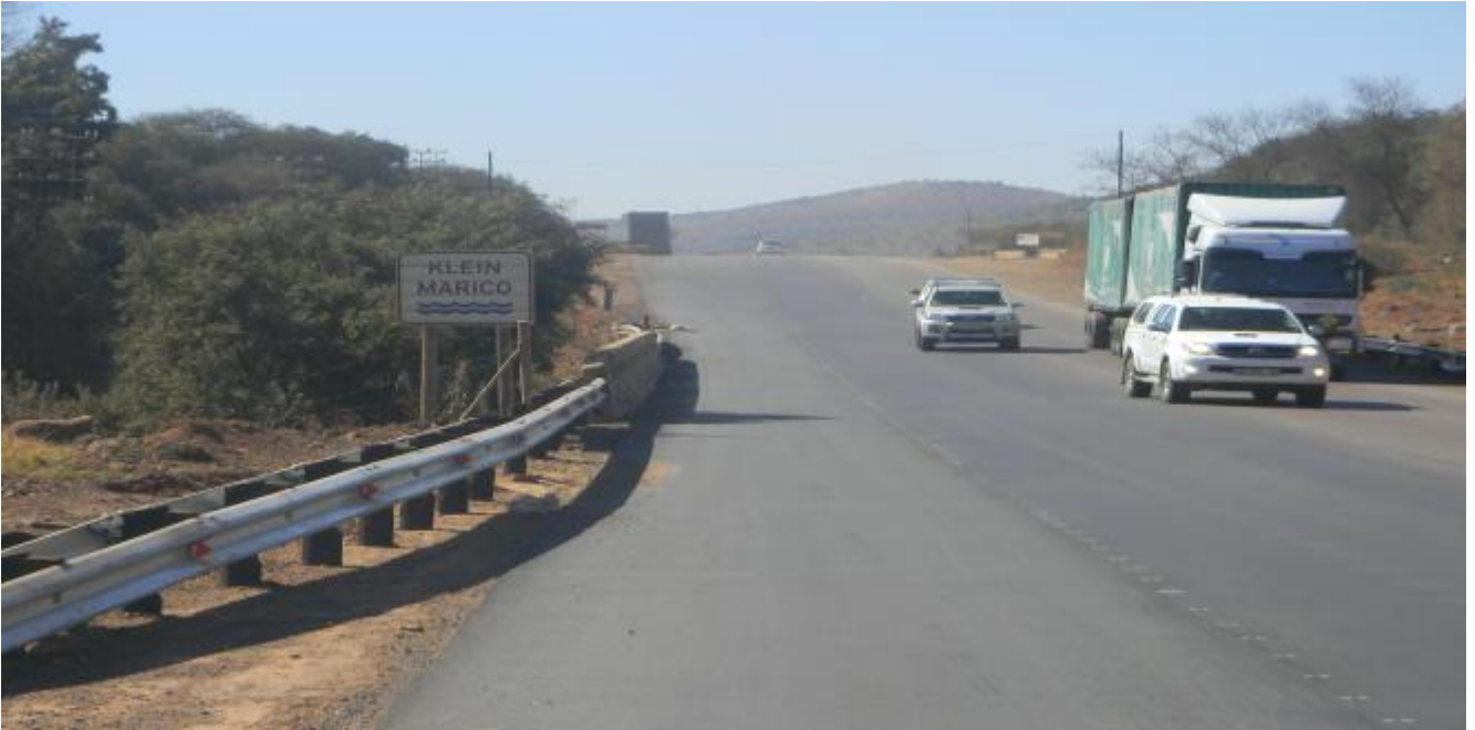
Plate 21: Photo 21: View of N4 Road and Klein Marico that marks the eastern boundary of the development site (Photograph © by Author 2016)
