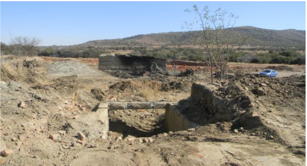
Plate 14: Photo 14: View of vandalized brick moulding infrastructure at the centre of the site (Photograph © by Author 2016)
