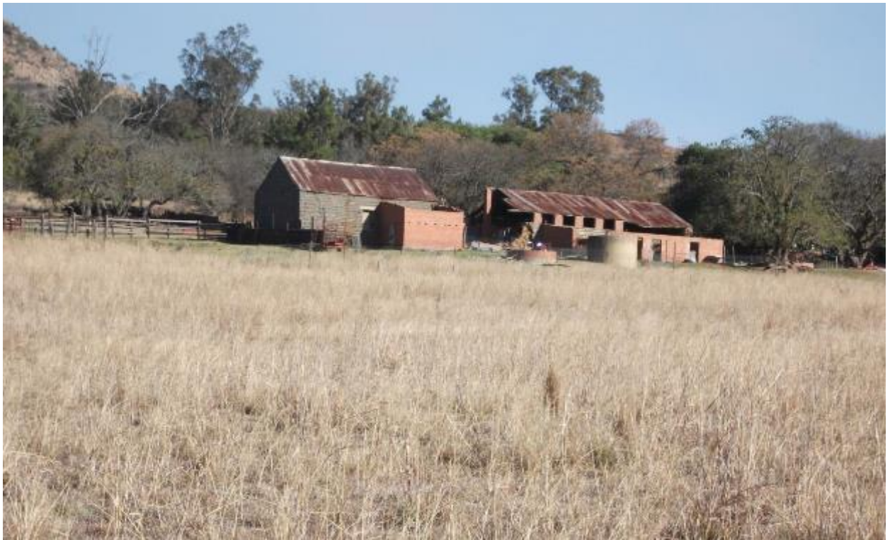
Figure 5: Structures older than 60 years
