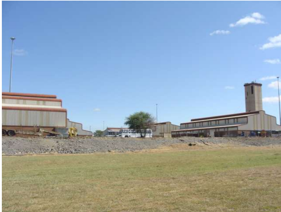
Figure 3 Some of the mine buildings in the surveyed area.
