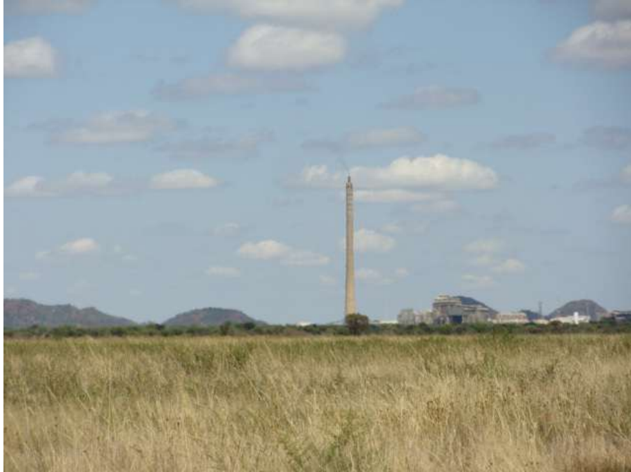
Figure 9 General view of the rehabilitated area with mining infrastructure in the background.
