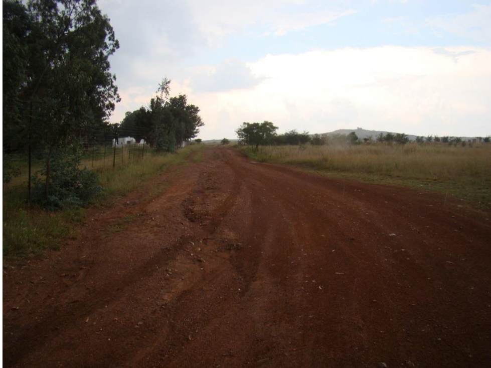
Fig. 9: The pipeline route facing east at the point where it changes direction from the south (at the tarred road, figs. 10 & 11), to east where the dirt road starts. The proposed line will be adjacent the fence.
