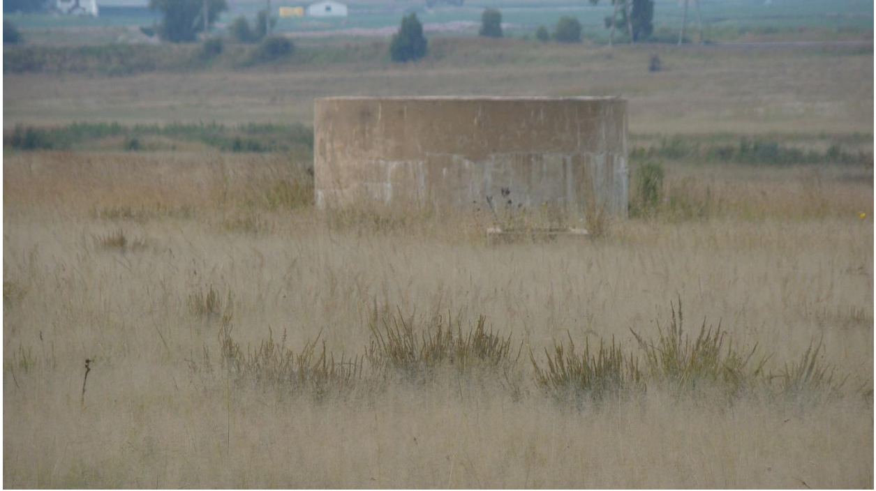
Fig. 15: The inlet or connection point, where the proposed pipeline will connect with the existing sewer line.
