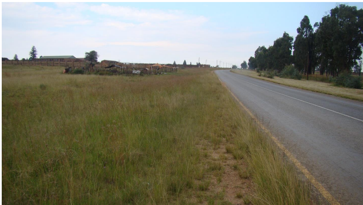
Fig. 10: The pipeline route will follow within the road reserve to the left or north of the tarred road.
