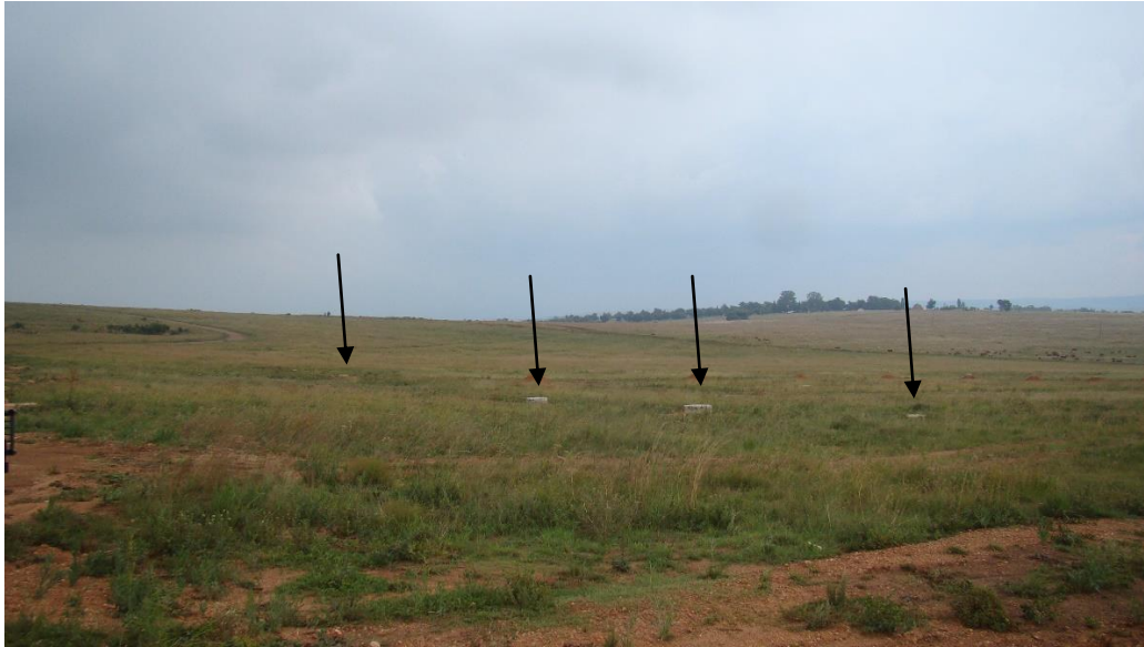
Fig. 1: A general view of the study area facing west. Some infrastructure has already been established for the Ridgeview development such as pipelines (arrows indicate the manholes), and a road network (see Fig. 18).
