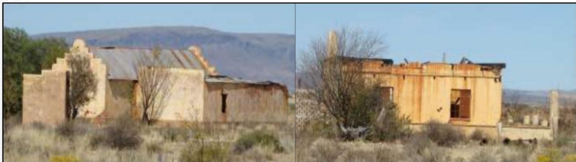
Figure 6-11: Views of vernacular farm houses and house ruins in the landscape (ACO Associates cc 2013).
