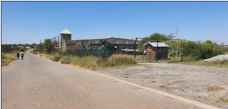
Figure 17: General view of the western section of the survey footprint
