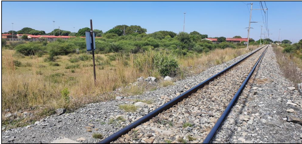
Figure 14: General view of the central section of the survey footprint (infrastructure)
