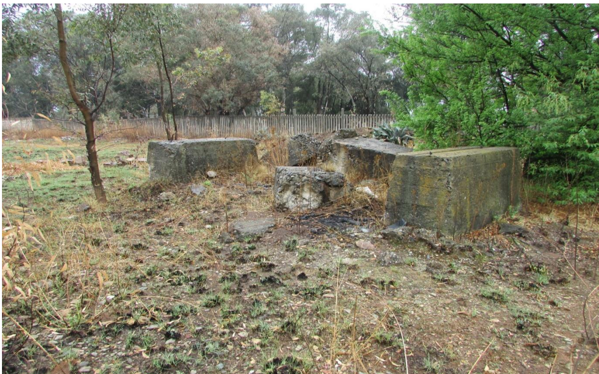
Figure 9: Blocks of concrete/cement in the Alternative 2 area. These were more than likely dumped here.
