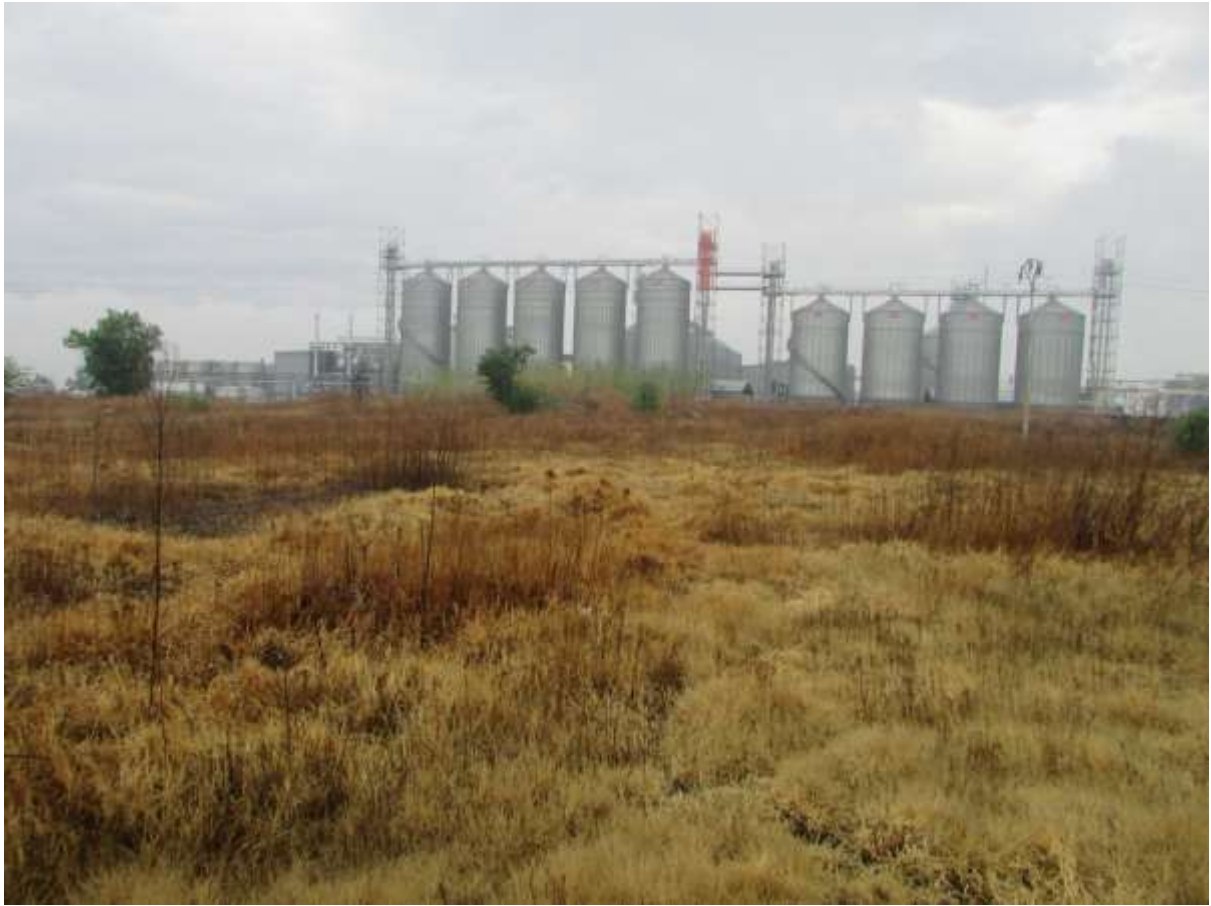
Figure 3: A general view of the Alternative 2 study area near Boksburg Unilever's plant.
