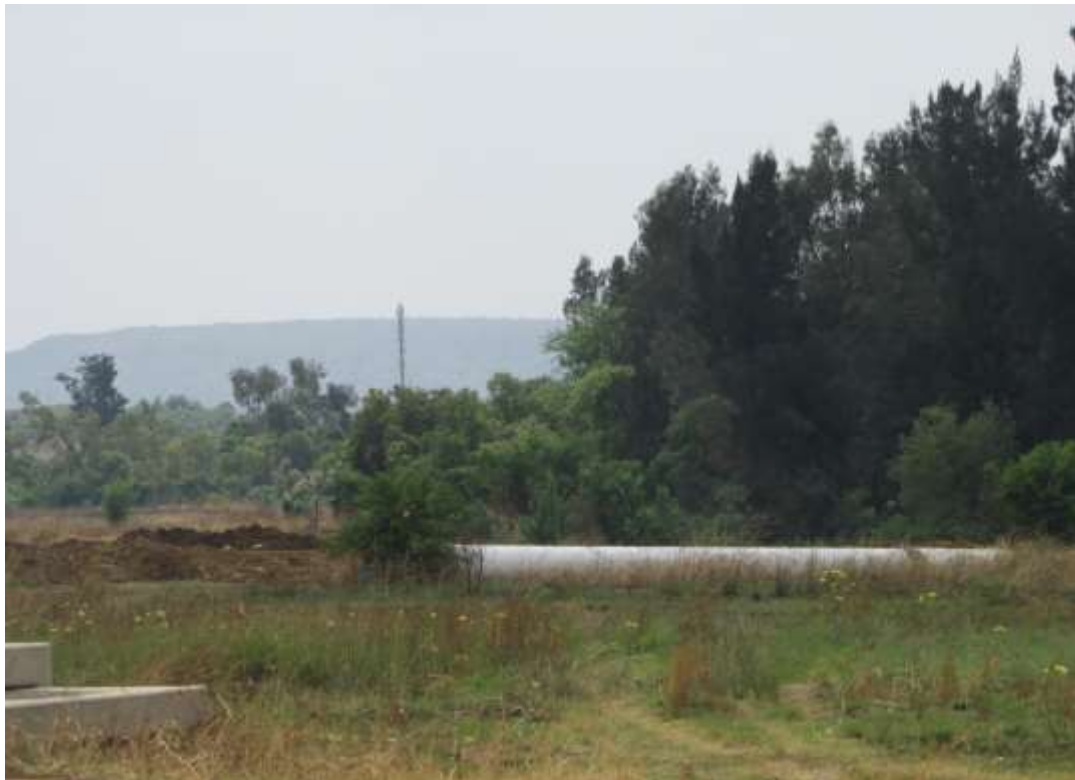
Figure 31: Another part of the Section B line towards Solomon Mahlangu Drive.
