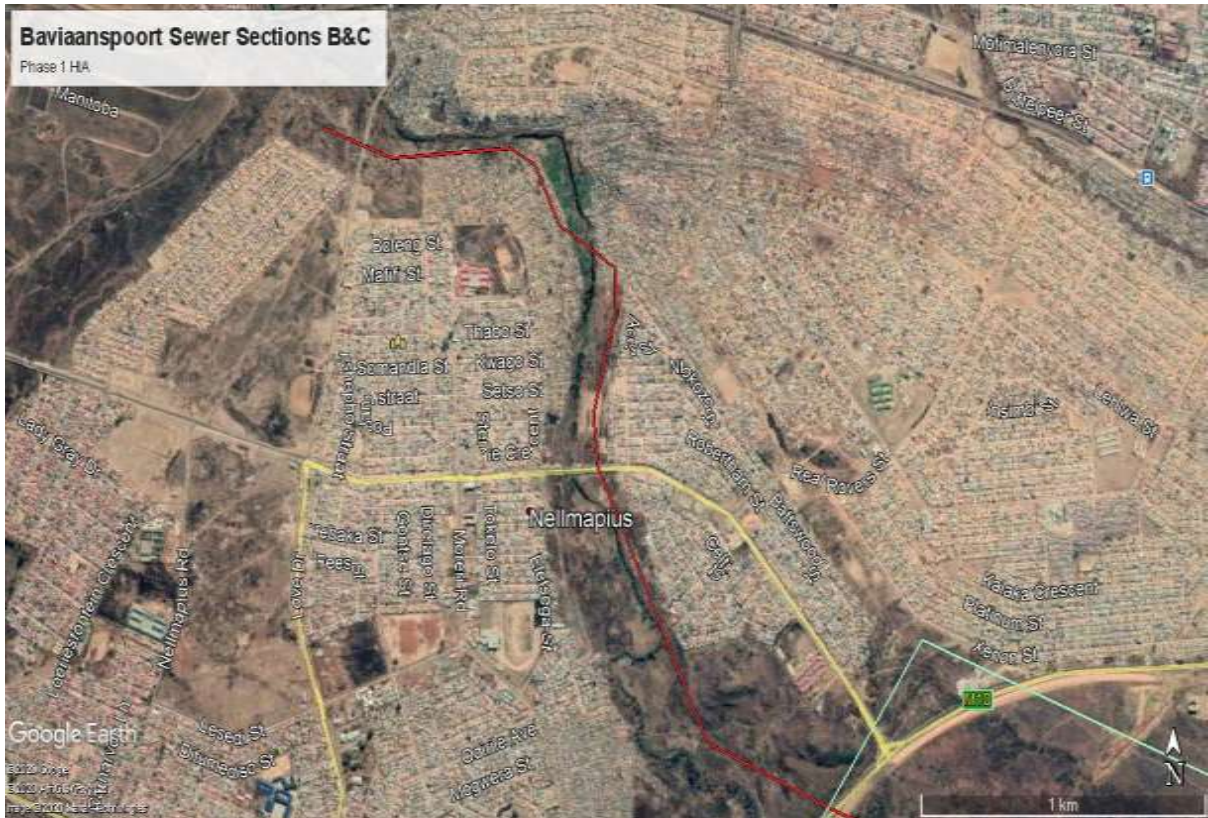
Figure 16: Aerial view of Section C line from Solomon Mahlangu Drive to Nellmapius. Large parts are located in and between informal and more formal urban settlements (Google Earth 2020).
