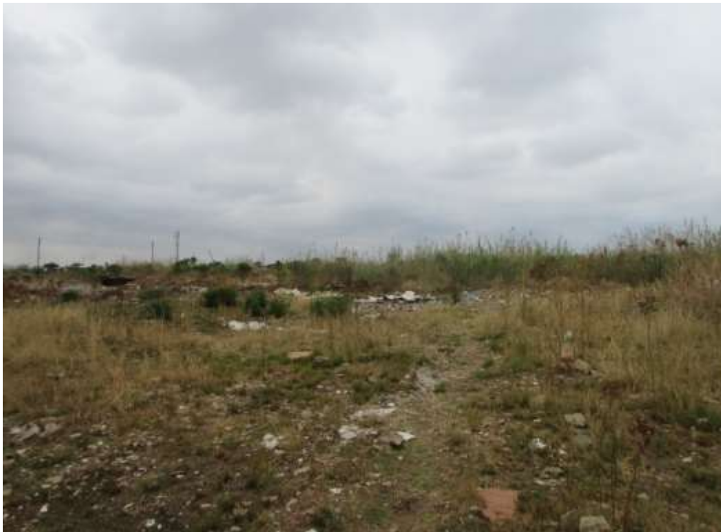
Figure 10: A view of the refuse dumping found all over the Section C portion of the line.
