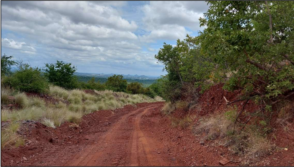
Figure 17: One of the roads associated with the study area.
