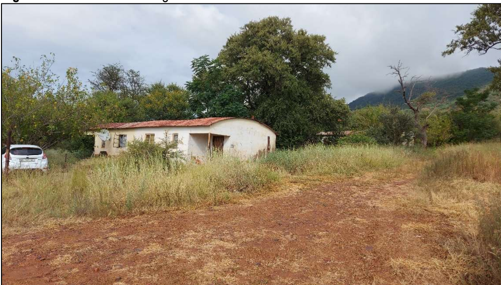
Figure 33: A remaining building at Site B03.
