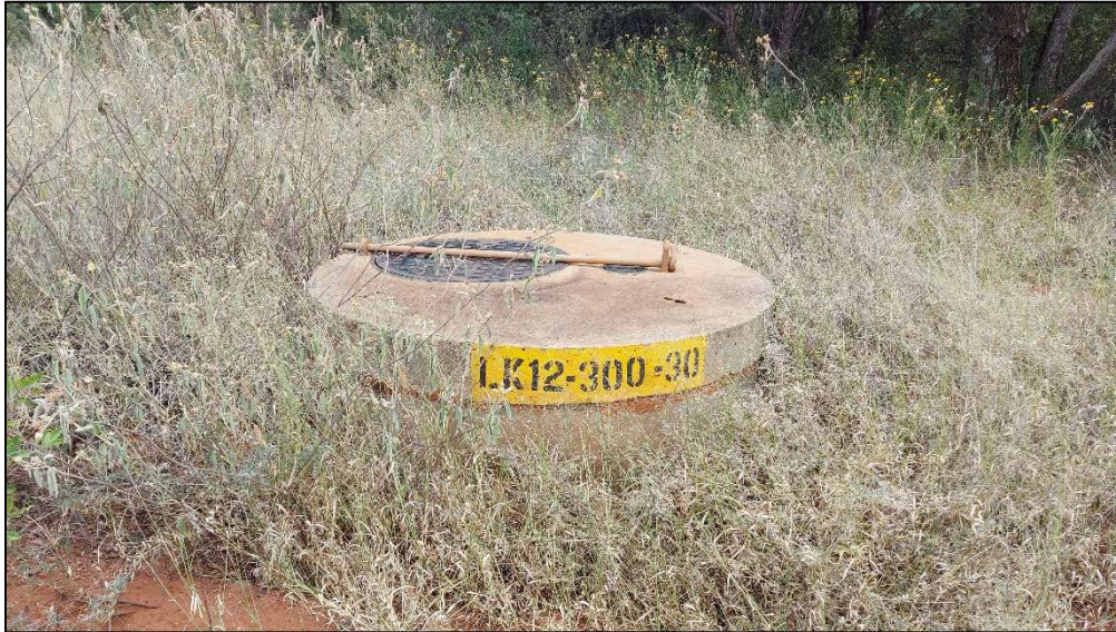
Figure 57: Cement and metal feature at Site F12.
