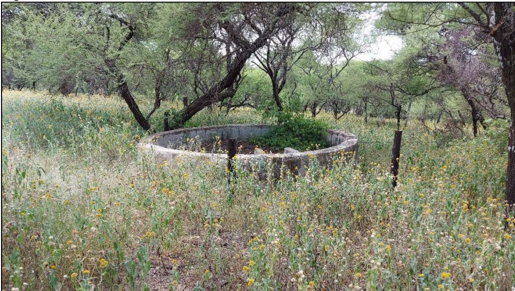
Figure 53: Small cement dam at Site B10.
