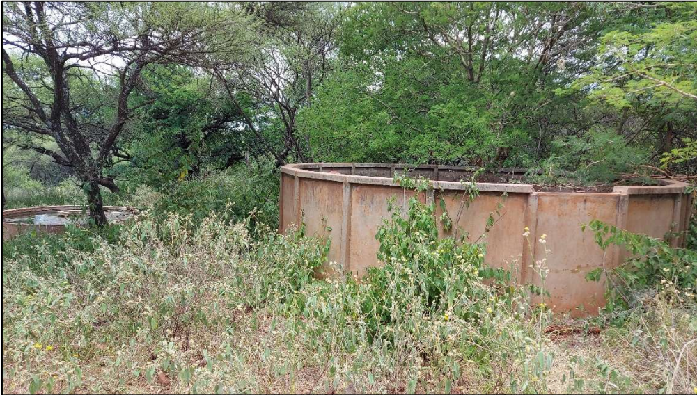
Figure 51: Cement dam at Site F09.
