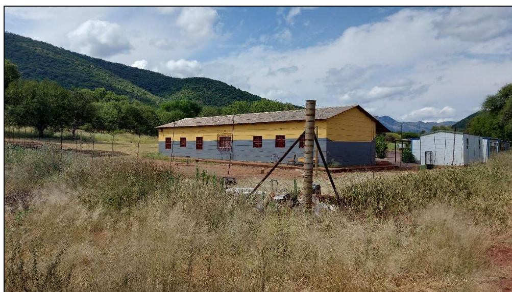
Figure 47: School at Site B04.
