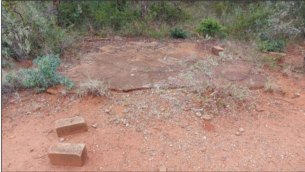
Figure 46: Building foundation / cement slab at Site F05.
