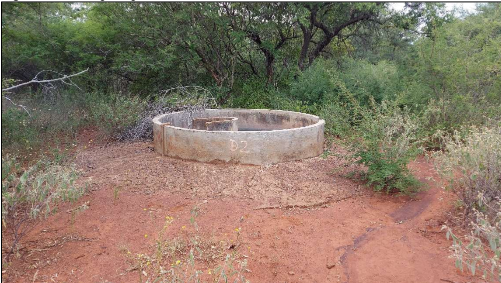
Figure 49: Cement dam at Site F07.
