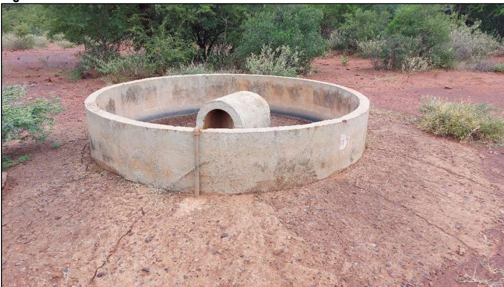
Figure 50: Cement dam at Site F08.
