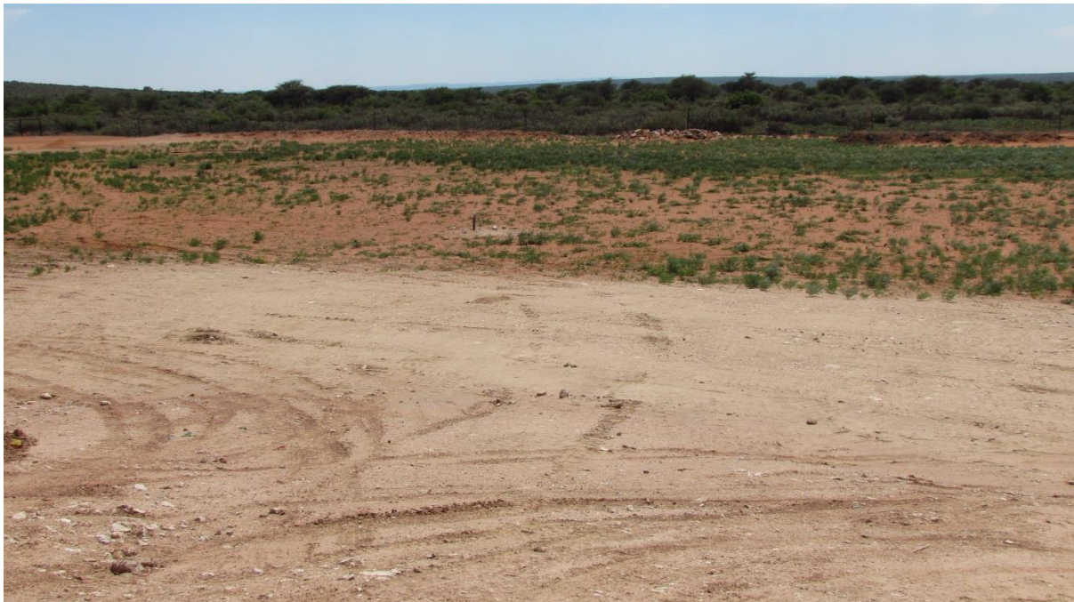
Topsoil removed to the surface of the calcrete immediately east of the Wastewater Treatment Works.
