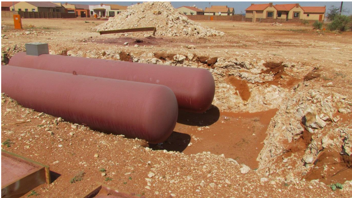
Parts of the gas reticulation at Bestwood Township Development (above and below): sunk into the top of the calcrete.
