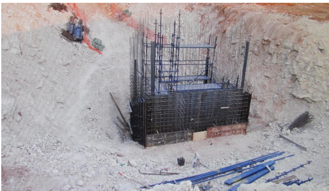
Photograph showing preparation for the construction of the Waterwater Treatment Works: shallow aeolian sands with subsurface calcrete formation (above), the latter (below), during construction of the Works, at least 11 m in thickness (F. Cawood pers.comm.). (Photos: Mr Fred Cawood)
