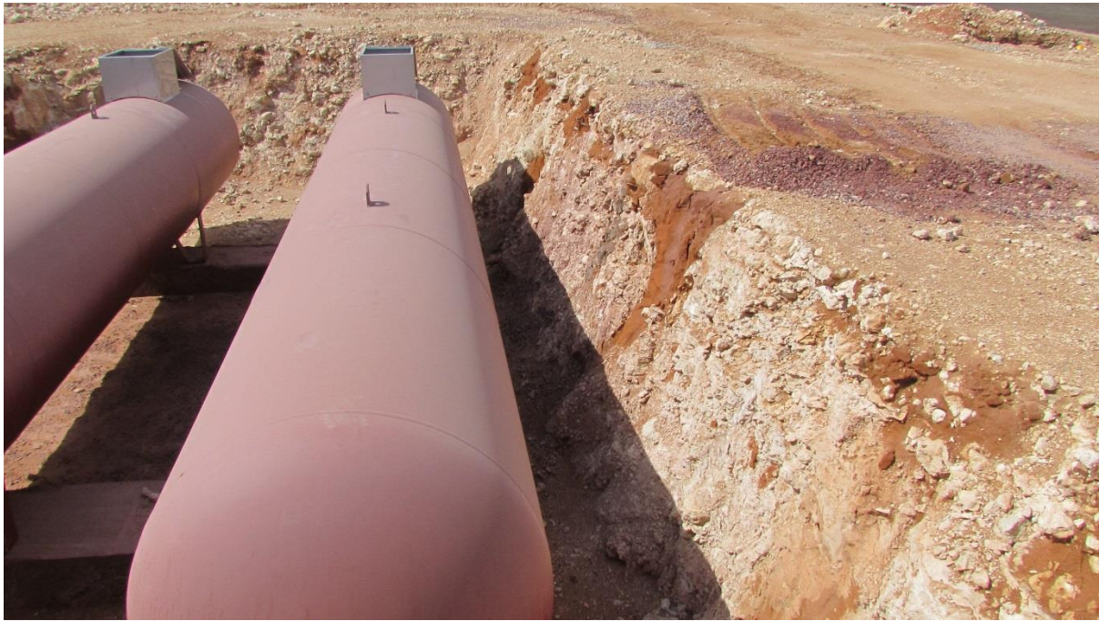
Parts of the gas reticulation at Bestwood Township Development (above and below): sunk into the top of the calcrete.
