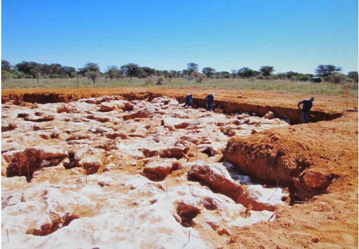
Photograph showing preparation for the construction of the Waterwater Treatment Works: shallow aeolian sands with subsurface calcrete formation (above), the latter (below), during construction of the Works, at least 11 m in thickness (F. Cawood pers.comm.). (Photos: Mr Fred Cawood)
