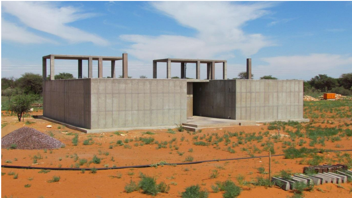
Completed Wastewater Sewage works at GPS position 292.
