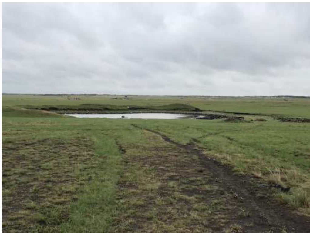
Figure 5: View of the earth dam within the site.
