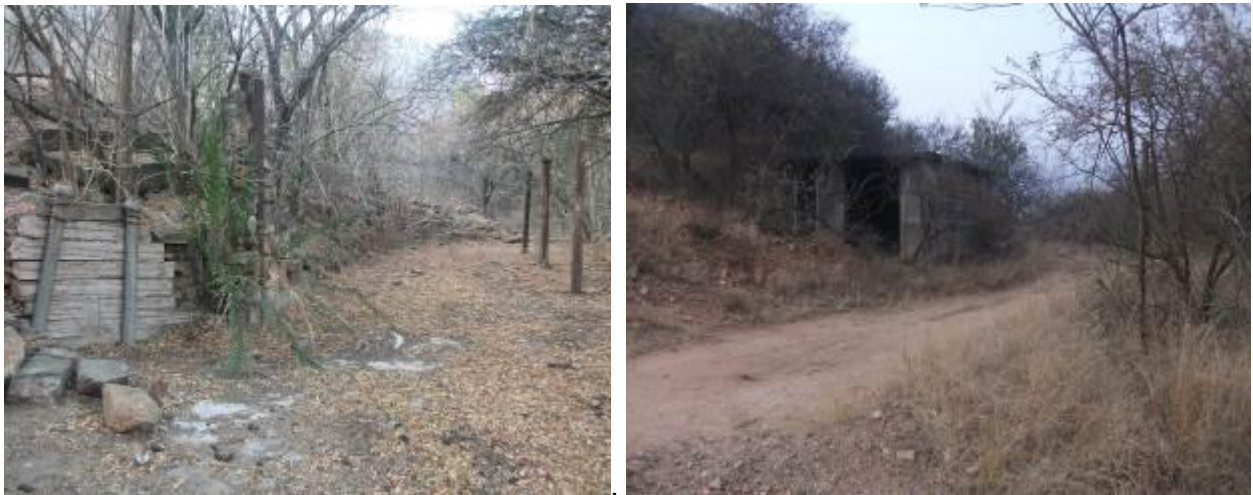
Figure 26: Remains of structures on river bank
