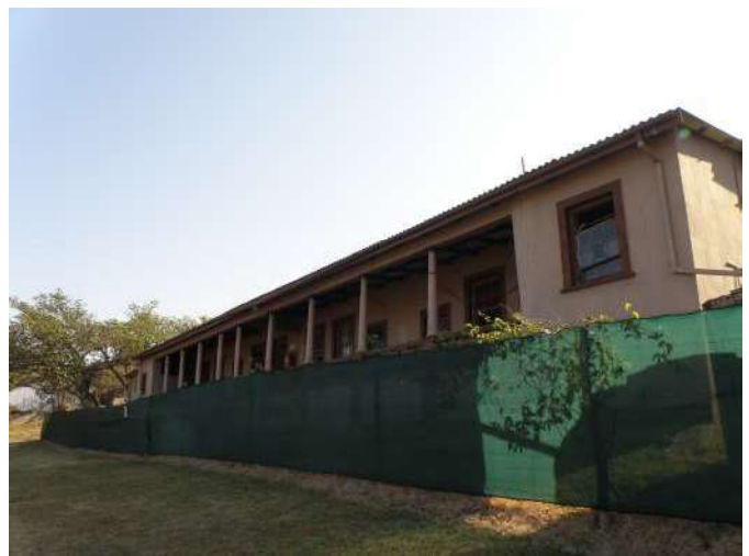
Figure 177: Building 1- Former School Building
