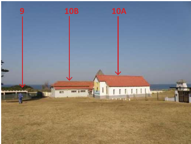
Figure 83: West elevation of old chapel
