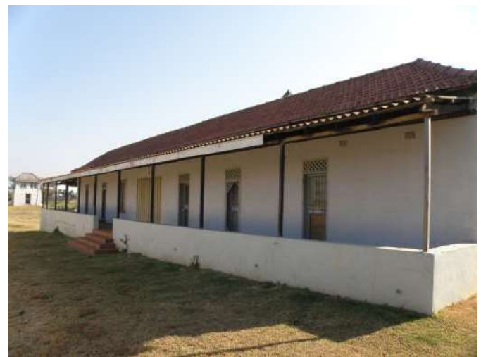
Figure 173: Building 10B - Accommodation
