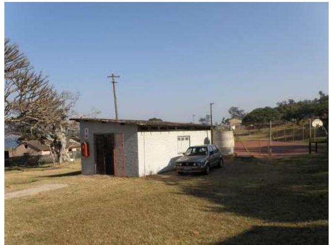
Figure 76: North West View
