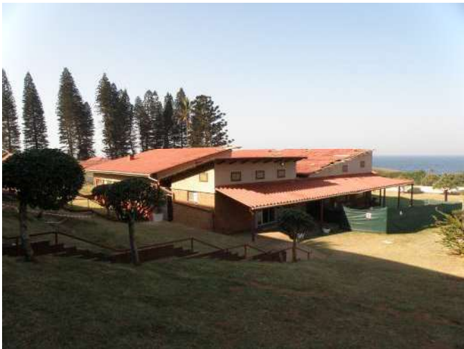
Figure 170: Building 7A & 7B - Dining Hall
