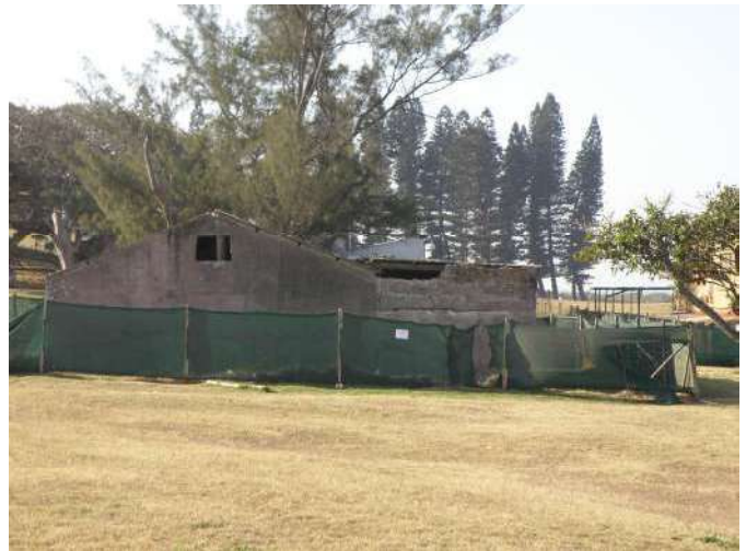
Figure 176: Building 11- Former Stable/Piggery/Dairy
