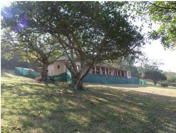
Figure 134: South East Elevation
