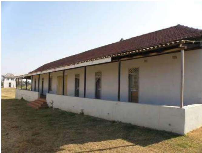
Figure 98: East elevation of 10B
