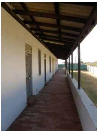
Figure 100: East elevation of 10B
