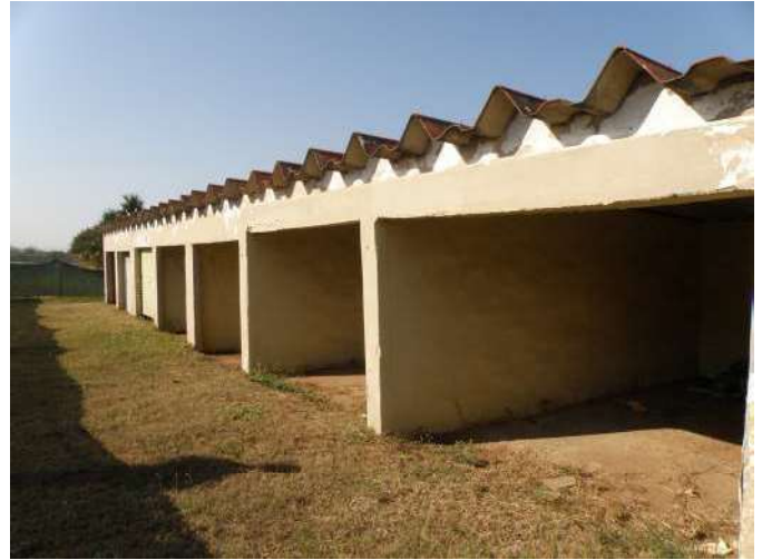
Figure 174: Building 9 - Old Garage
