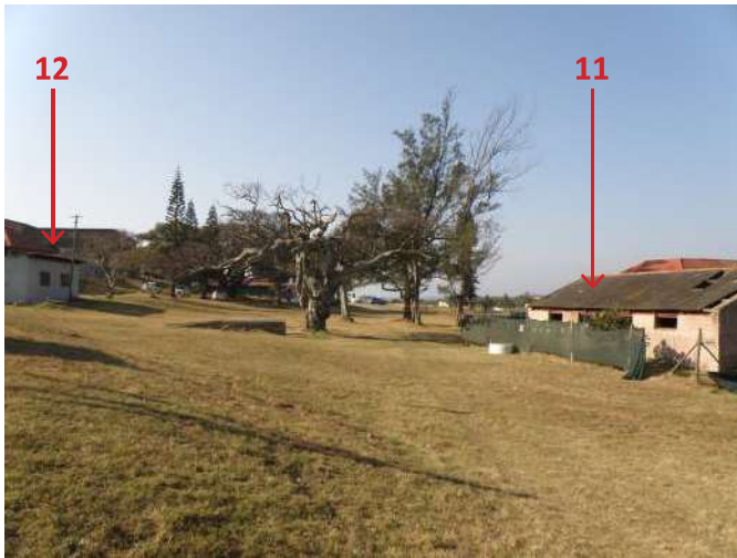
Figure 75: Looking north between buildings 12 and 11
