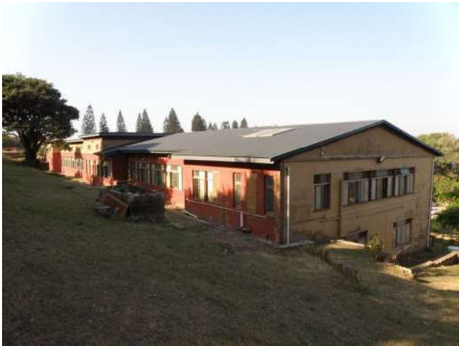
Figure 11: South West Corner
