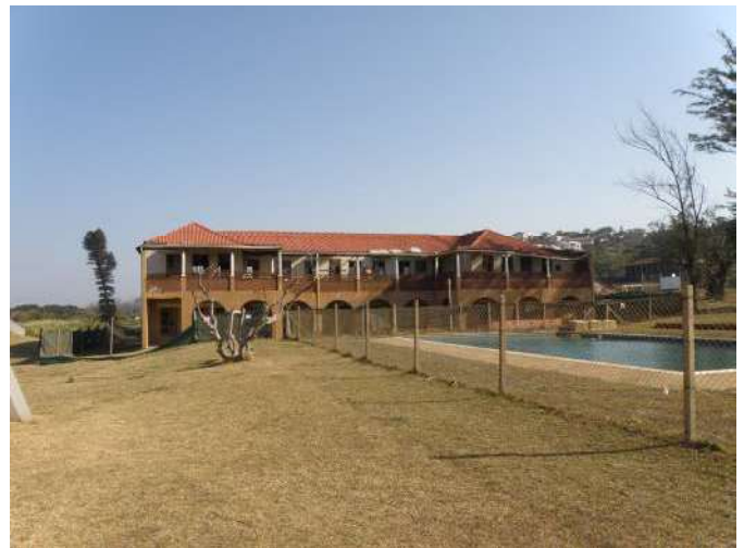
Figure 175: Building 13 - St. Vincent's, Old School Building
