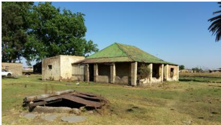
Figure 3-2: Dilapidated structure (FH15)
