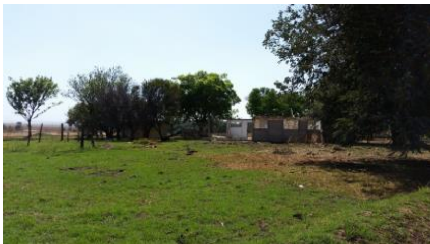
Figure 3-3: Abandoned structure (FH12)
