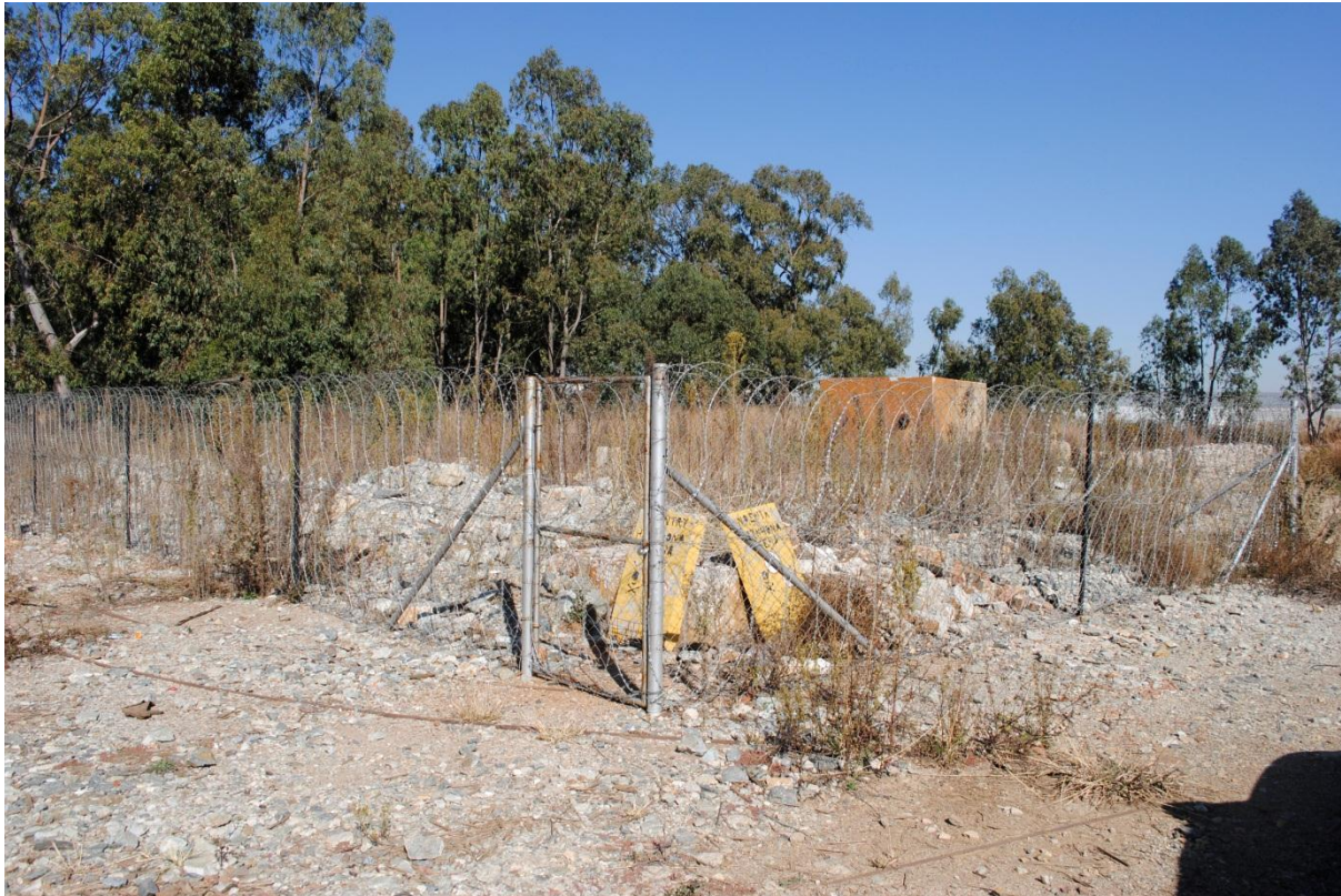
Figure 1: At the proposed abstraction point all infrastructure has been demolished and removed. This was the location of the old head gear
