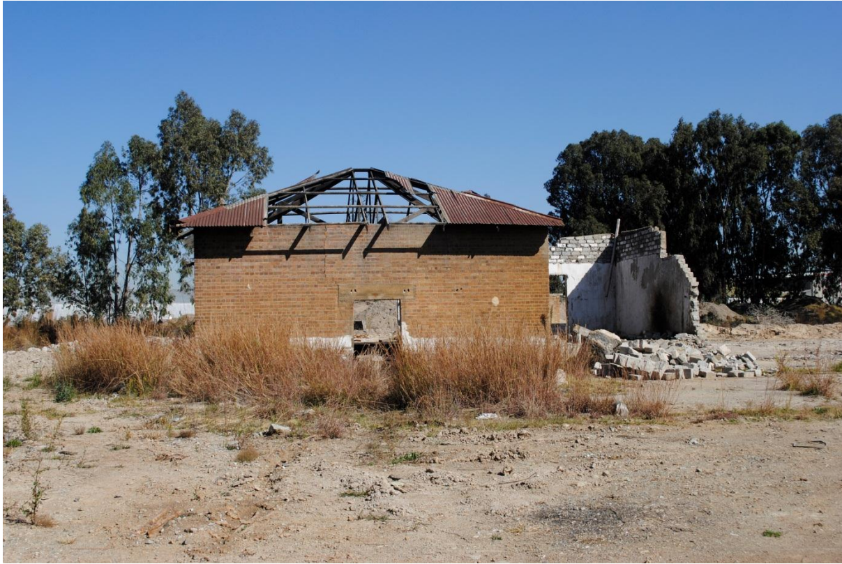
Figure 2: Only building still existing on the proposed abstraction property
