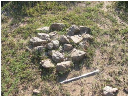
Figure 1-16: A single grain bin foundation next to an old agricultural field.
