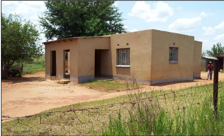
Figure 2: Occupied house in the region of the survey area
