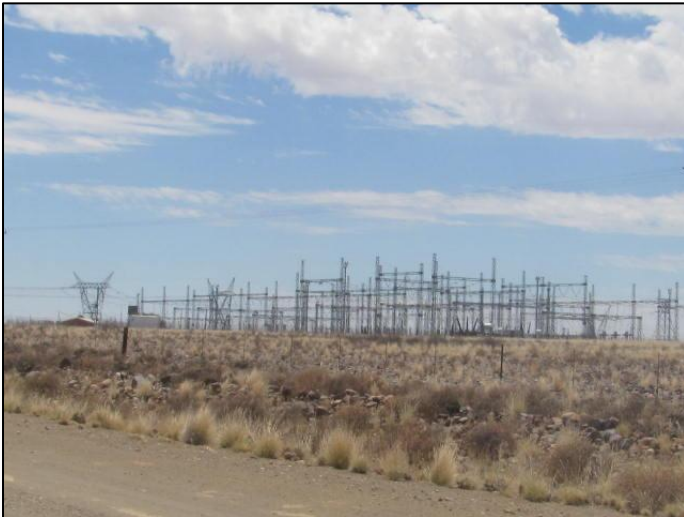
Figure 4: Aries substation 1 km south of the study area
