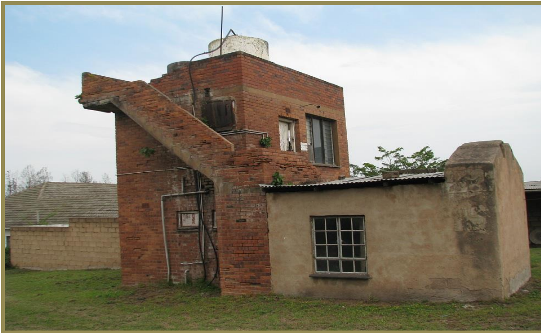
FIGURE 3. RED-BRICK WATER TOWER
