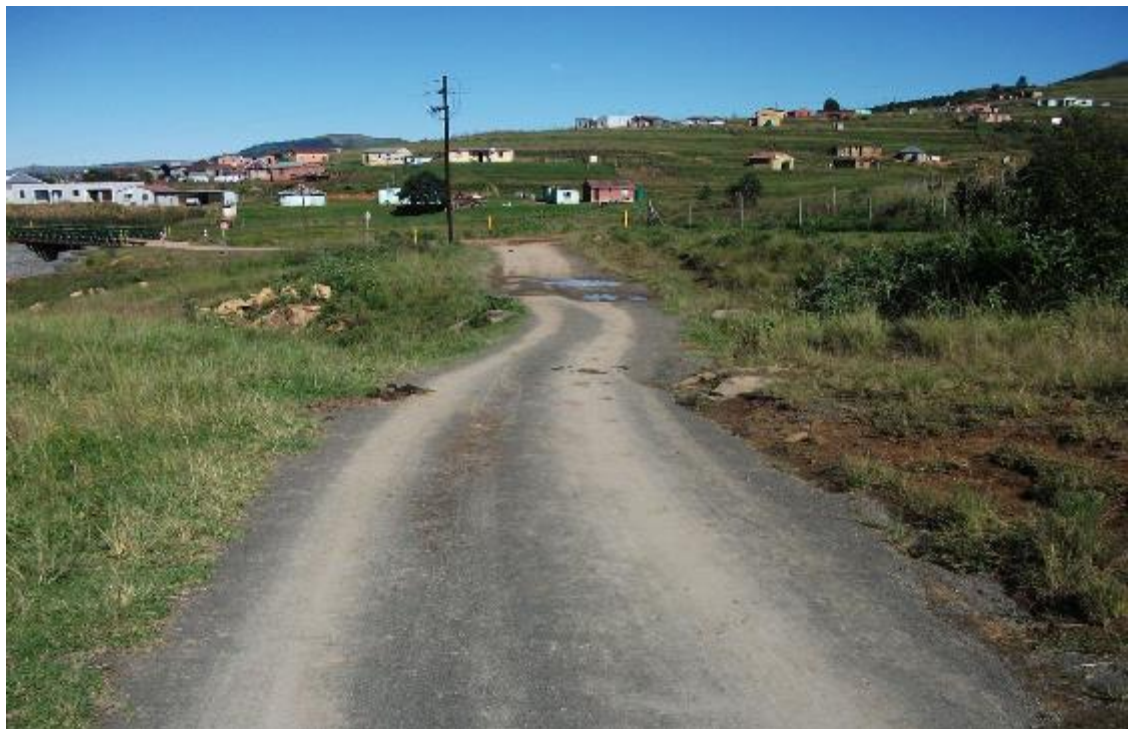
Figure 15: Northern end of Baleni Road looking in a south-westerly direction
