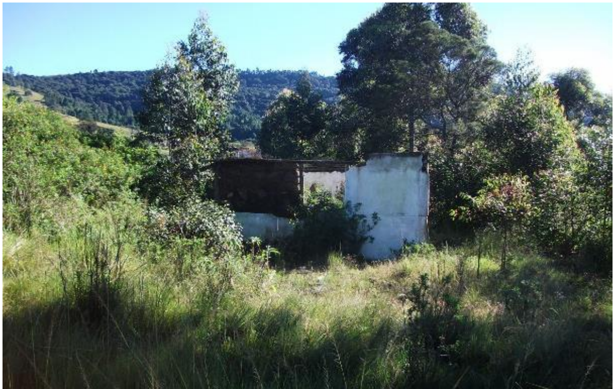
Figure 11: Abandoned structure to east of Baleni Road
