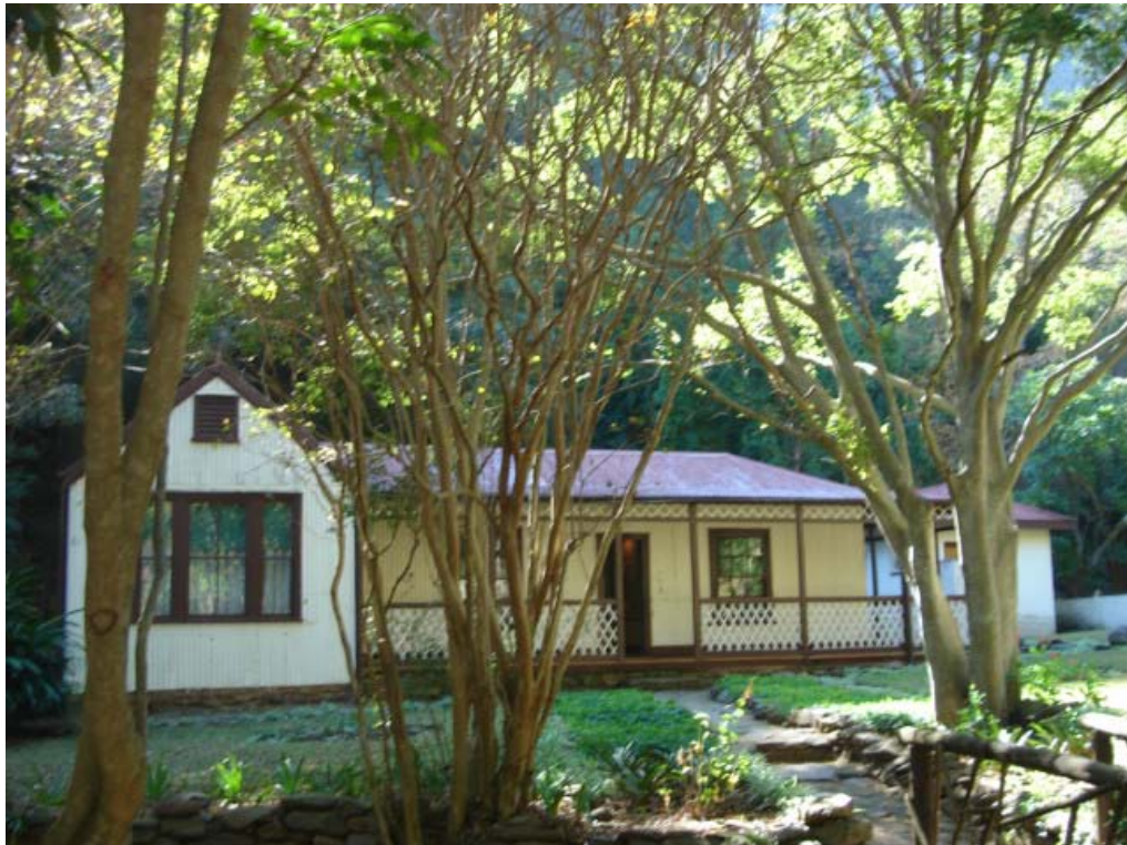
No. 6 Fernlea House in Rimers Creek
