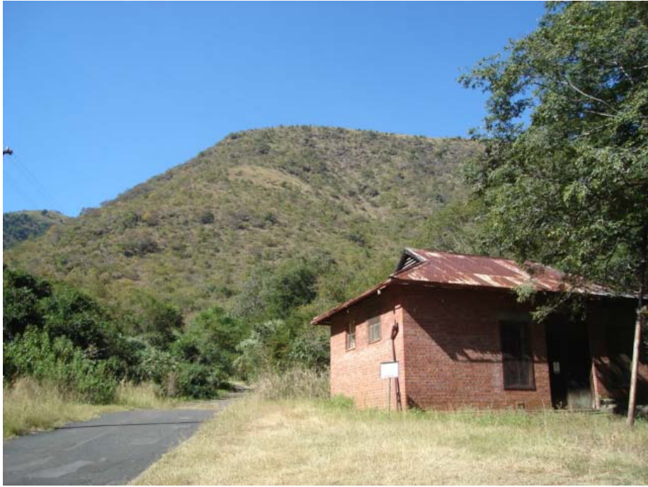
No. 7 Turbine Building in Rimers Creek
