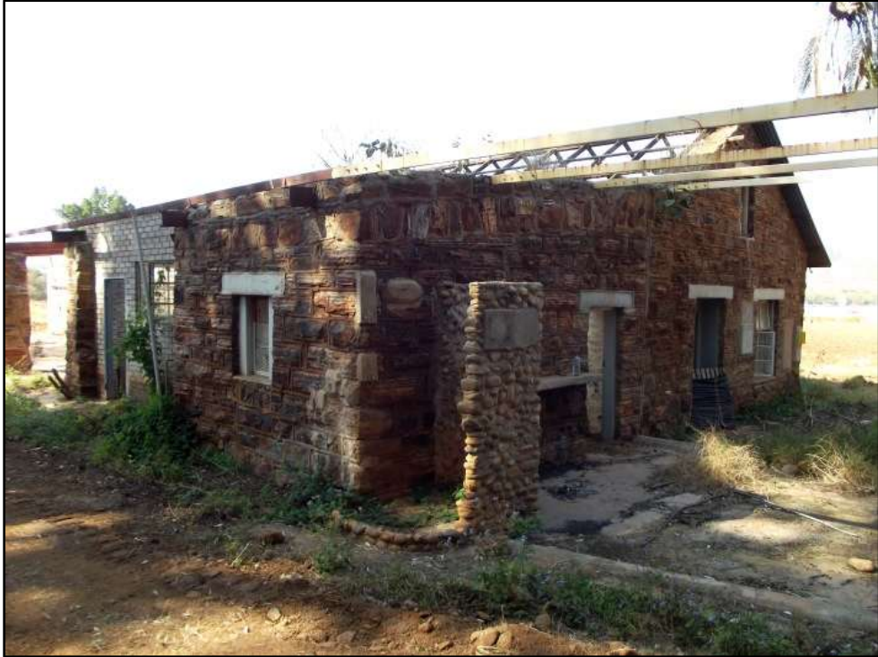
Fig. 87. Site BV 4. Photo taken in north eastern direction.
