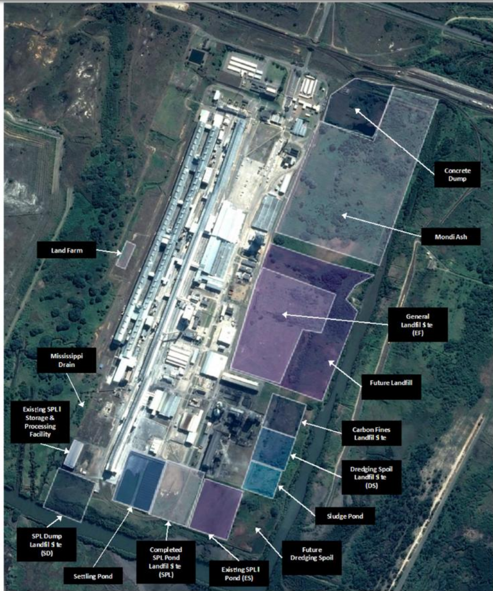
Figure 2: Aerial view of the Bayside Smelter in Richards Bay, highlighting the locations of all of the legacy 'landfill' areas.
