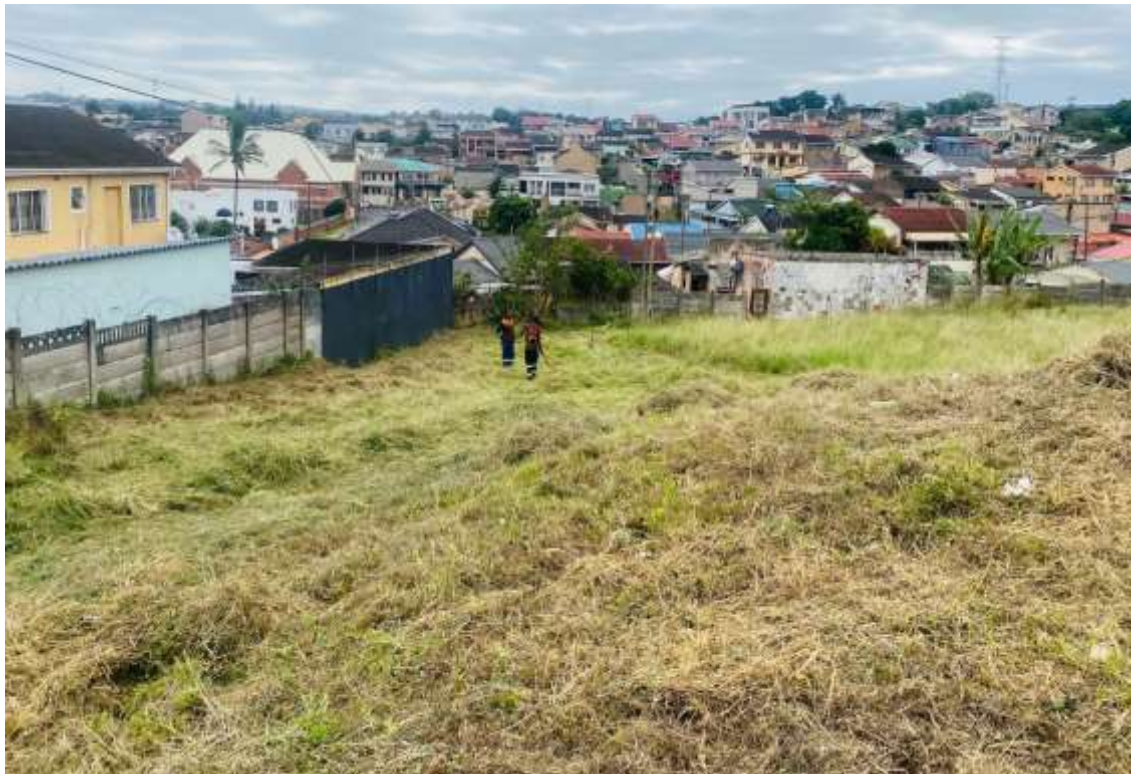
Figure 7: Grass cutting on project site
