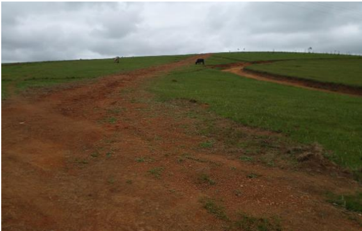
Figure 6: Newly installed pipeline next to gravel road en-route to reservoir
