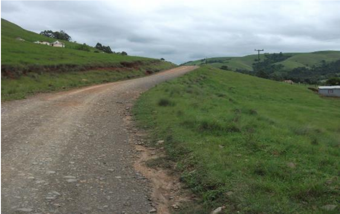
Figure 10: Pipeline route with dwellings situated some distance from road
