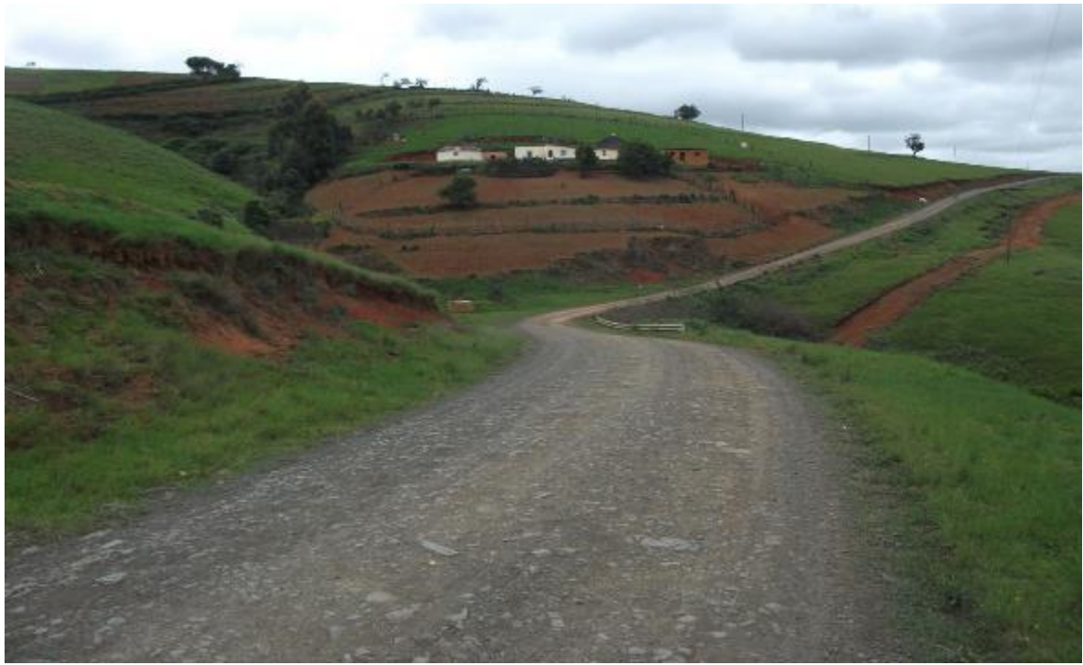
Figure 12: Steep topography and newly installed pipeline route
