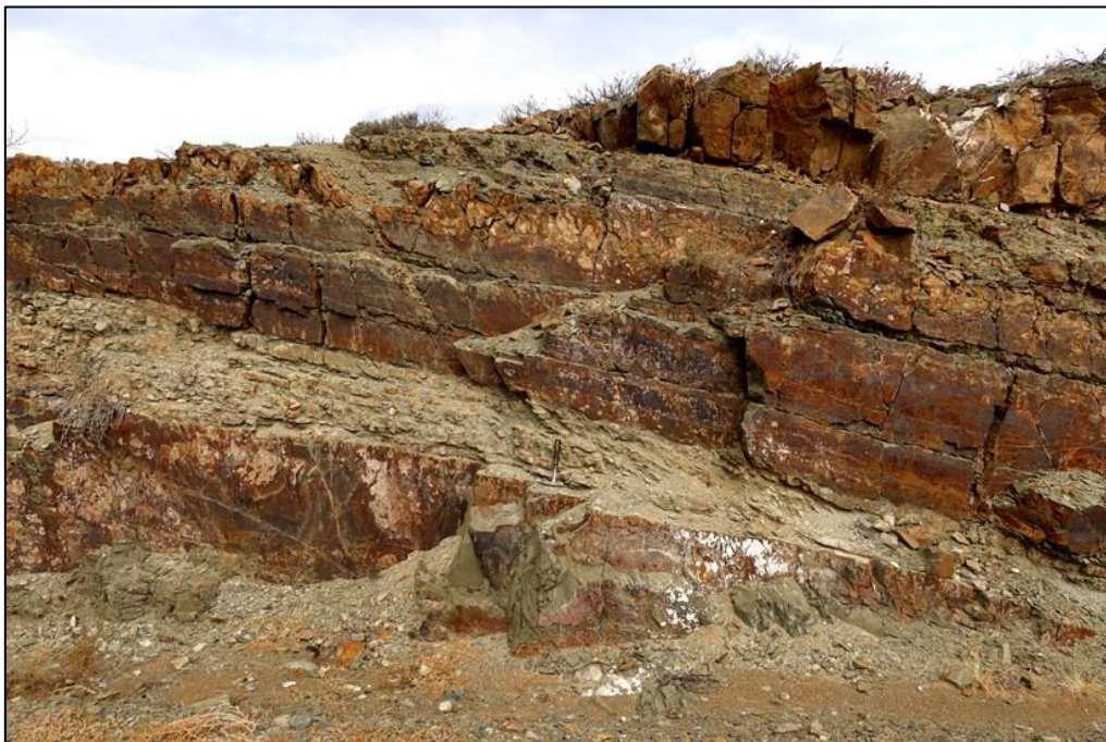
Figure 23: Low-angle thrust marked by pale, bedding-parallel, highly-brecciated zone of bedrock (at level of hammer, 30 cm long), N12 road cutting through the Abrahamskraal Formation just west of the WEF project area, (Loc. 055). Thrusting has been from the south and is often associated with large-scale quartz veining (Figure 24).
