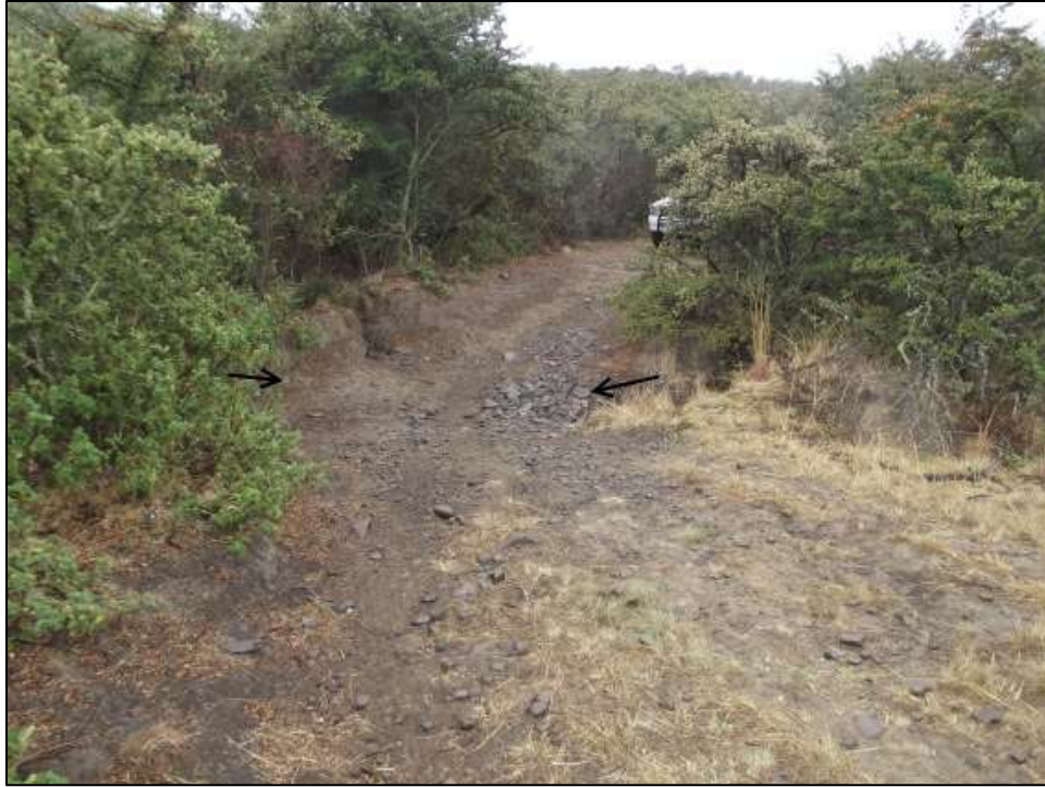
Fig. 18. Site WB 8. A general view of the small bridge. Photo taken in northern direction.
