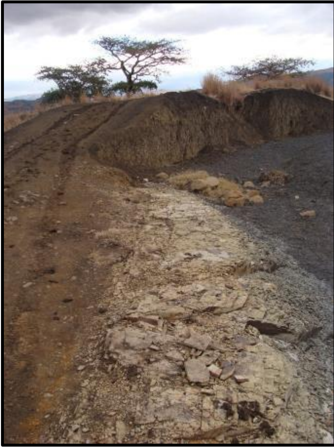
Figure 9: Point 1, (“Watercourse”) depicting the existing road running over bedrock in the form of fossiliferous Beaufort mudstone. This is the approximate place where the causeway will be positioned. Looking up the valley in a northerly direction
